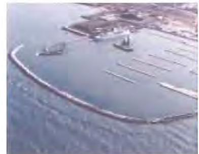
The core of the protective breakwater at the Hammond Marina (Hammond, Ind.) consists of 65,000 tons of ACBF slag. After extensive testing, Indiana's Department of Environmental Management approved ACBF slag as an acceptable product for use in Lake Michigan.
