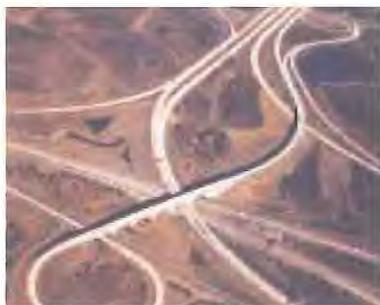
M-5/I-96 concrete interchange, Farmington Hills, MI. Used ACBF slag for open grade drainage course and concrete pavement.
