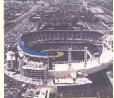
The new Comiskey Park (Chicago, IL) contains over 900,000 lightweight concrete block, used EXPANDED BLAST FURNACE SLAG AGGREGATE in order to achieve the desired weight, as well as fire resistance requirements.
