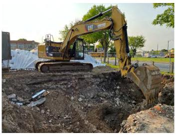
**Photo No. 24** Excavation of Soils Beneath the Former USTs
