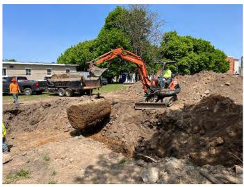
Photo No. 11 Removal of UST-05 (UST-06 & 07 Pictured on Trailer)
