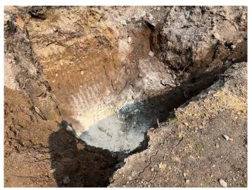
Photo No. 27 ORC Powder Installed Beneath Former UST-03 & 04
