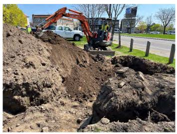
Photo No. 4 Excavator Uncovering UST-05 through 07
