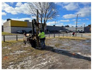
Photo No. 3 Geoprobe Setup at GP-06
