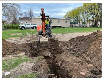
Photo No. 2 Fill-port of UST-02 Identified During Excavation
