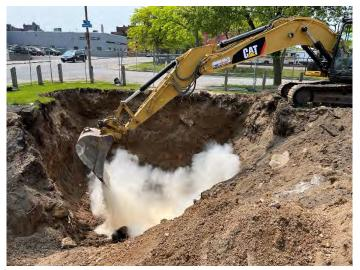
Photo No. 29 ORC Installed in Southwest Corner of the Excavation
