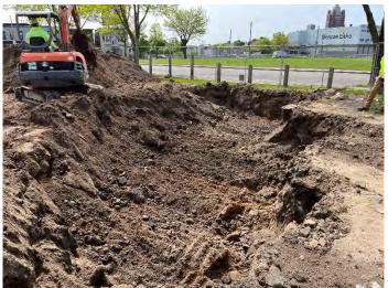
Photo No. 3 Excavation and Stockpiling of Clean Overburden
