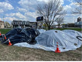
Photo No. 6 Final Imported Soil Stockpile
