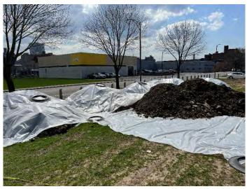
Photo No. 5 Stockpiling of Imported Soils from CVMF
