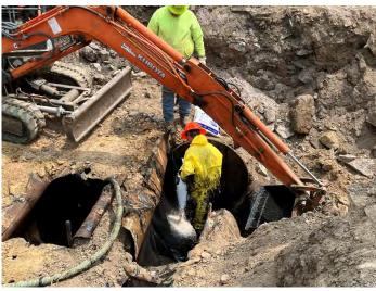
Photo No. 14 Interior Cleaning of UST-04 (UST-03 Pictured Left)
