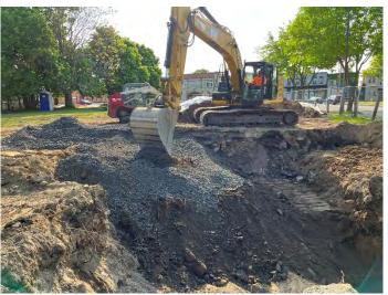
Photo No. 31 Excavation Backfill and Surface Restoration Process
