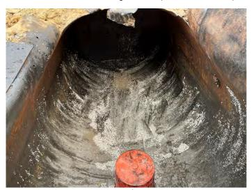
Photo No. 16 UST-03 After Interior Cleaning
