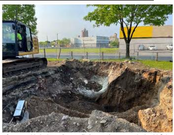
Photo No. 26 ORC Powder Installed Beneath Former UST-05, 06 & 07
