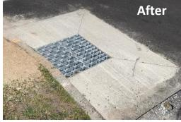
Note: Collars are only installed when an adjustment is necessary due to structural condition, frame & grate condition, elevation issues or for a new catch basin.
