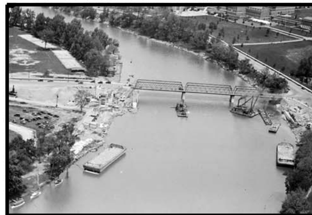
VIEW OF PARK AND OLD BRIDGE
