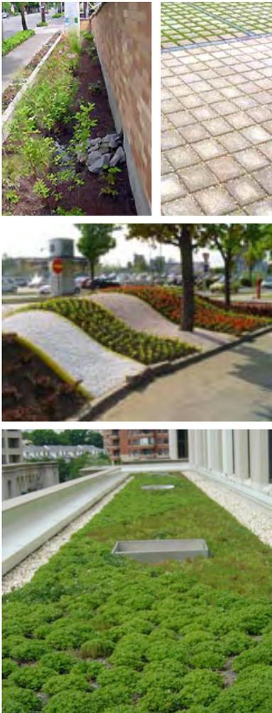
Examples of green development - pervious paving, swales and green roofs.
