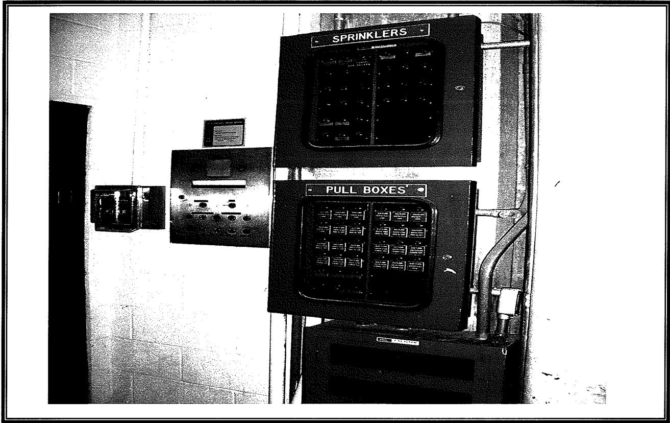
Photo 3 Photo Date 12/05/06 Non-addressibel fire alarm system Midtown Tower
