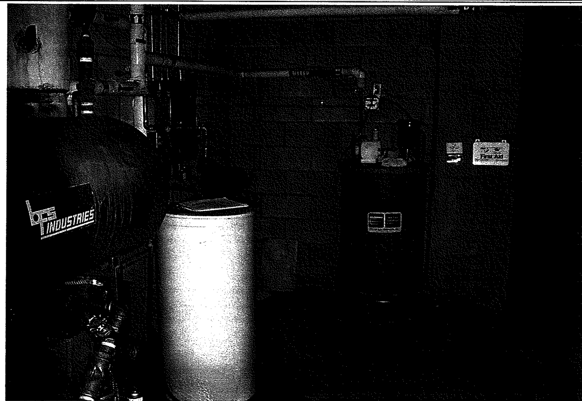
Photo 4 View of the boiler room in the McCurdy's Building. Photo Date 11/21/06 Containers of chemical treatment for the boiler system.
