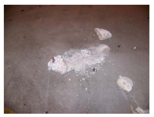
4. Level A: Debonding in Traffic Membrane & Deterioration in Concrete Overlay
