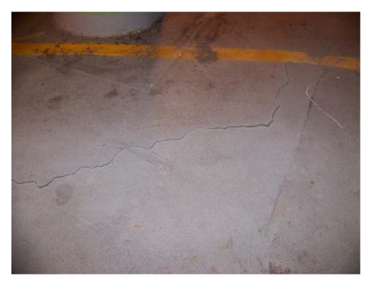
3. Level A: Crack in Traffic Membrane
