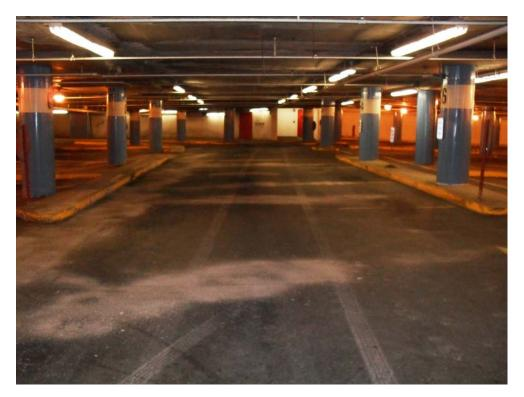
17. Level C: Ceiling Scaling Deposits on Main Drive Aisle
