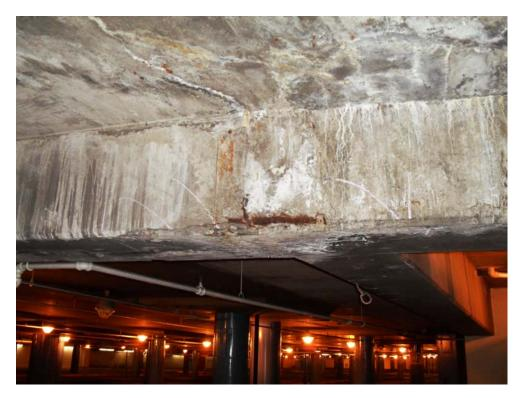
20. Level C: Ceiling and Beam Deterioration
