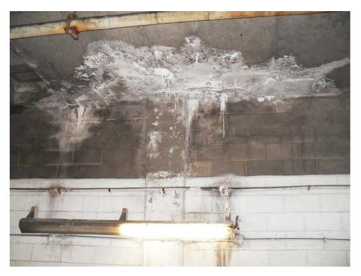
44. Exit to Court Street: Ceiling Deterioration and Column Cracking
