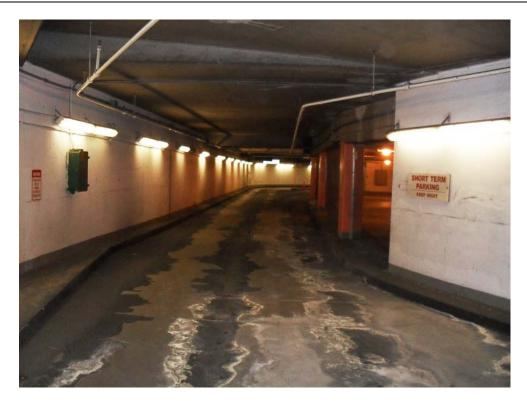
7. Level B: Worn Traffic Membrane in Recirculation Aisle
