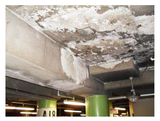
10. Level A: Ceiling and Beam Deterioration
