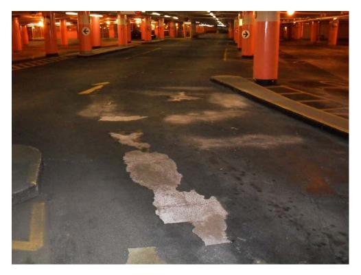
6. Level B: Transverse Crack in Exposed Concrete Overlay
