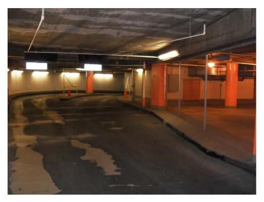
8. Level B: Worn Traffic Membrane in Recirculation Aisle
