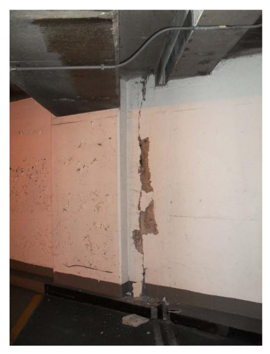
31. Level B: Wall Crack and Spall at Expansion Joint
