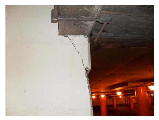
33. Level B: Diagonal Crack and Spall Under Beam at Stair S-9
