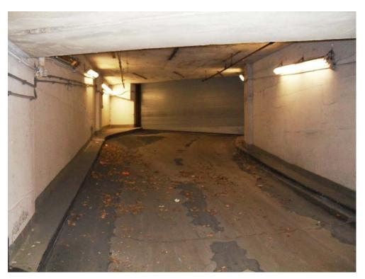
46. Broad Street Exit: Worn Traffic Membrane and Transverse Floor Crack
