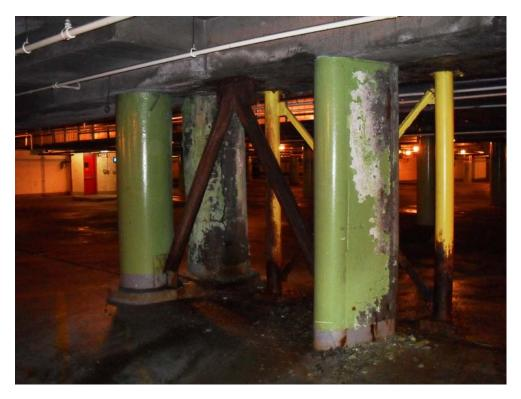
24. Level A: Columns 5-H and 5.4-H.1 Deterioration at Leaking Expansion Joint
