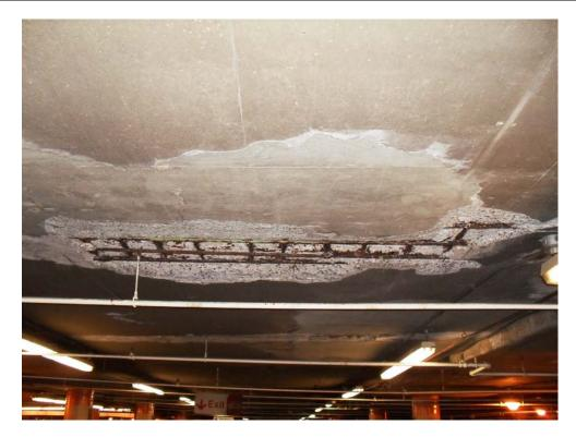
14. Level B: Ceiling Deterioration Adjacent to Previous Patch
