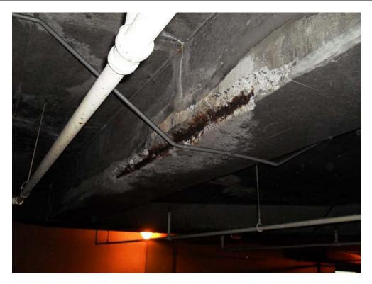
12. Level A: Beam Bottom Deterioration
