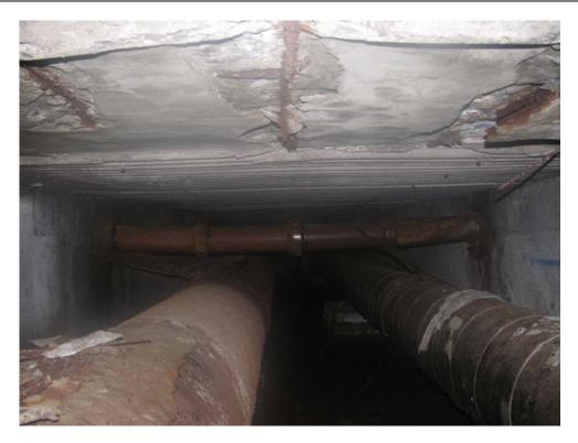
47. Level C: Utility Tunnel Roof Slab Deterioration
