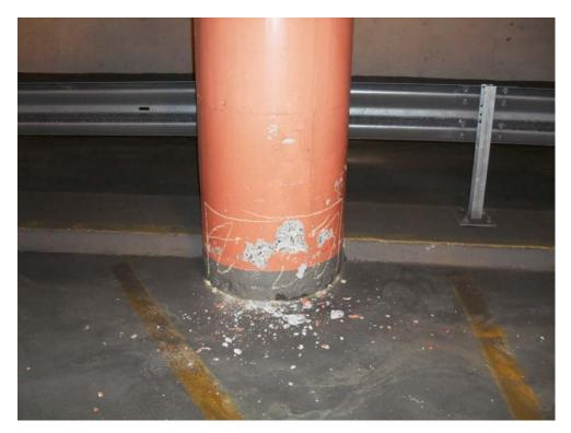
22. Level B: Typical Deterioration at Column Base
