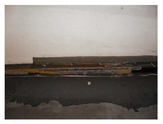
35. Level B: Curb Spall with Exposed Rebar
