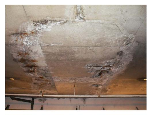
21. Level C: Ceiling Deterioration Around Previous Patch
