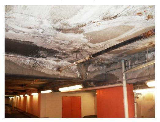
15. Level B: Ceiling Deterioration
