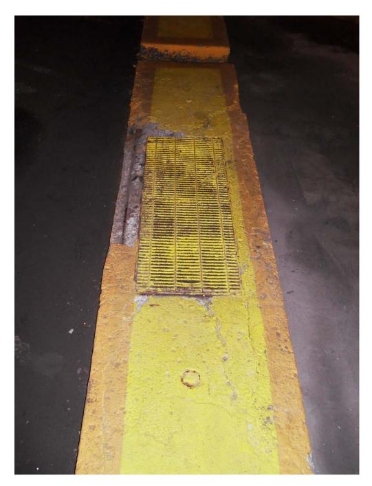
38. Level C: Typical Curb Scaling and Spall at Ventilation Grill
