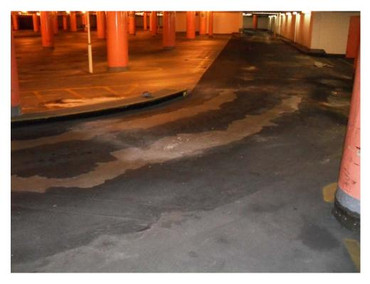
5. Level B: Worn Traffic Membrane and Ceiling Scaling Deposits on Floor
