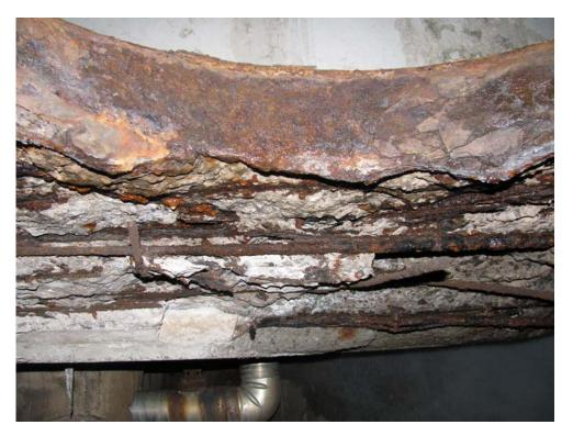
48. Level C: Utility Tunnel Roof Slab Deterioration
