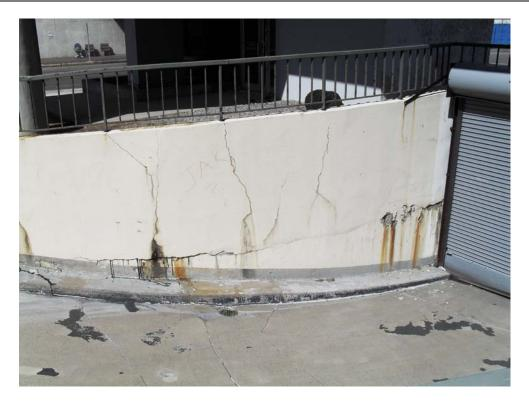
45. Broad Street Exit: Retaining Wall Cracks at Railing Posts
