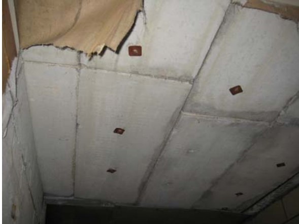
IMG 1655 – duct insulation blocks
