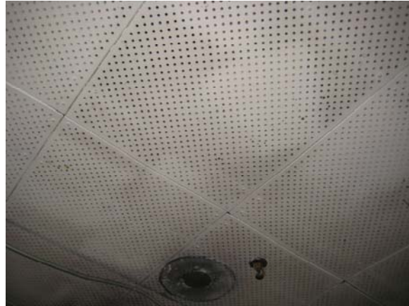
ACM Transite ceiling panels in basement
