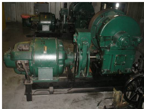
Elevator penthouse motor
