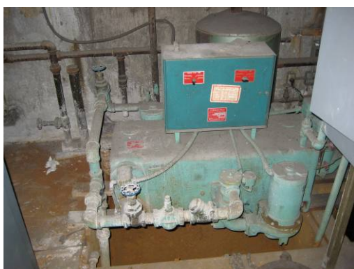
Oil-filled vacuum pump basement of B. Forman
