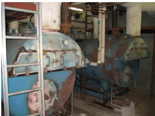
Boilers in boiler room
