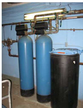
Water softener in Boiler Room
