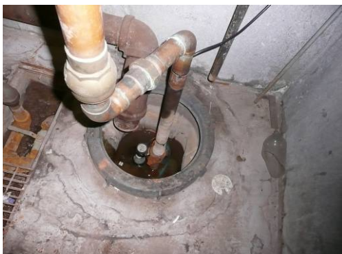
Sump in sub-basement of McCurdy's Building
