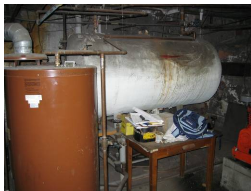
ACM wrapped water tank basement in B. Forman Building
