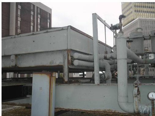
Cooling tower on roof
