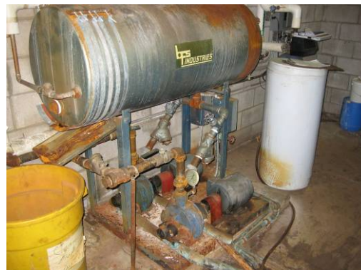
Descaling agent tank in boiler room
