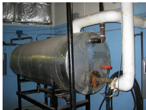
Expansion tank in boiler room
