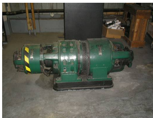
Oil filled motor - elevator penthouse
