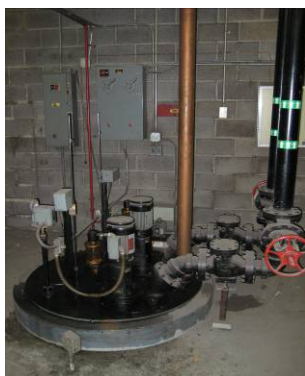
Sump pit and pumps to sewer in the northwest end of mechanical area
