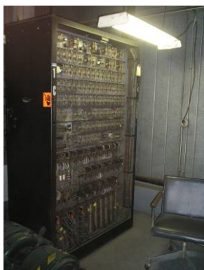
Elevator penthouse panel w/ capacitors
