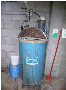
Descaler mixing tank Sub-basement of McCurdy's
