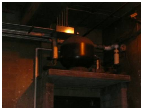
Compressor in underground service tunnel
