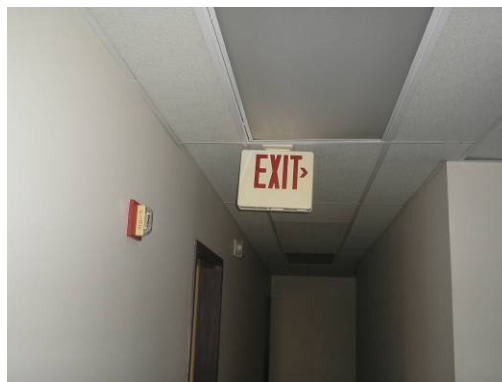
Emergency lighting and Exit sign on 4 th Floor
