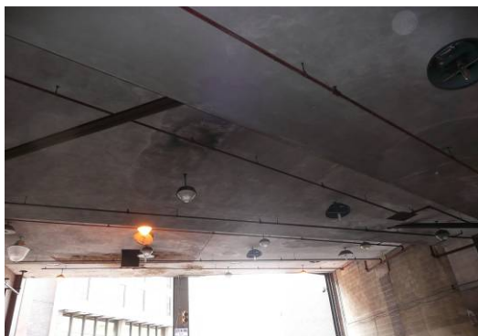
Mercury lamps at underground service tunnel entrance
