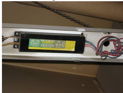
Light ballast in basement
