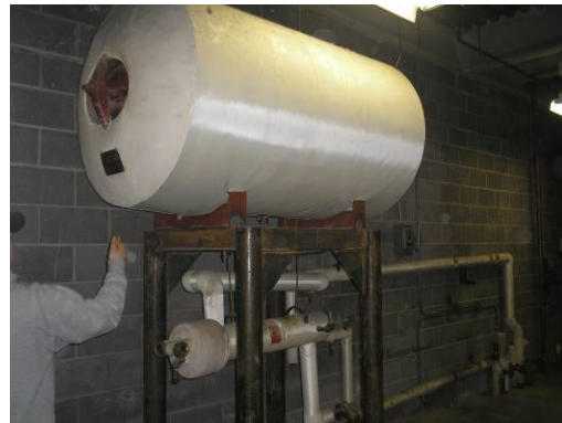
Hot water tank in elevator penthouse
