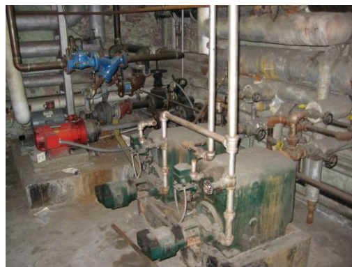
Oil filled vacuum pump in mechanical room
