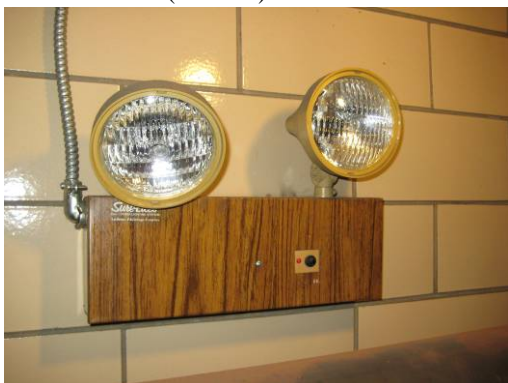
Emergency lighting in boiler room
