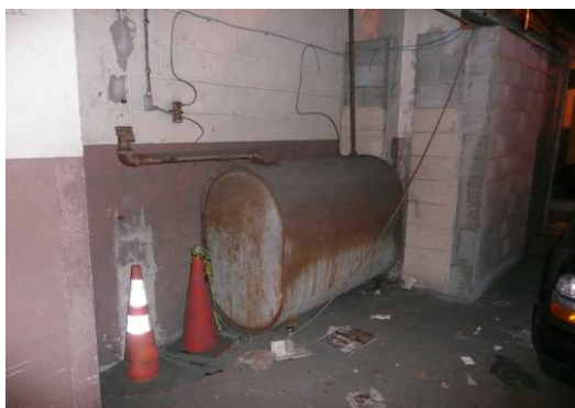
Generator AST at underground service tunnel near McCurdy's Building
