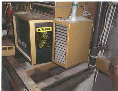
Natural gas generator in basement
