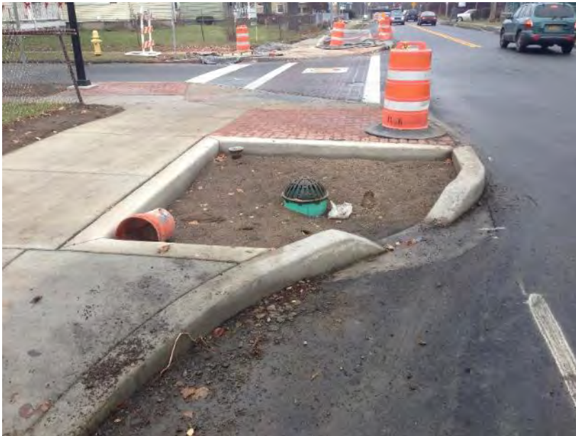
Example raingarden in bump out from North Union Street currently under construction
