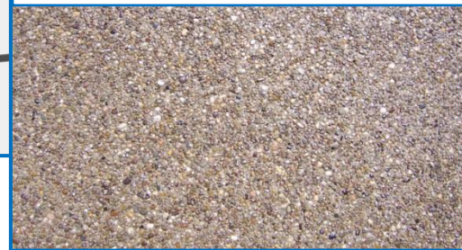
Exposed Aggregate Concrete Goodman Street at University
