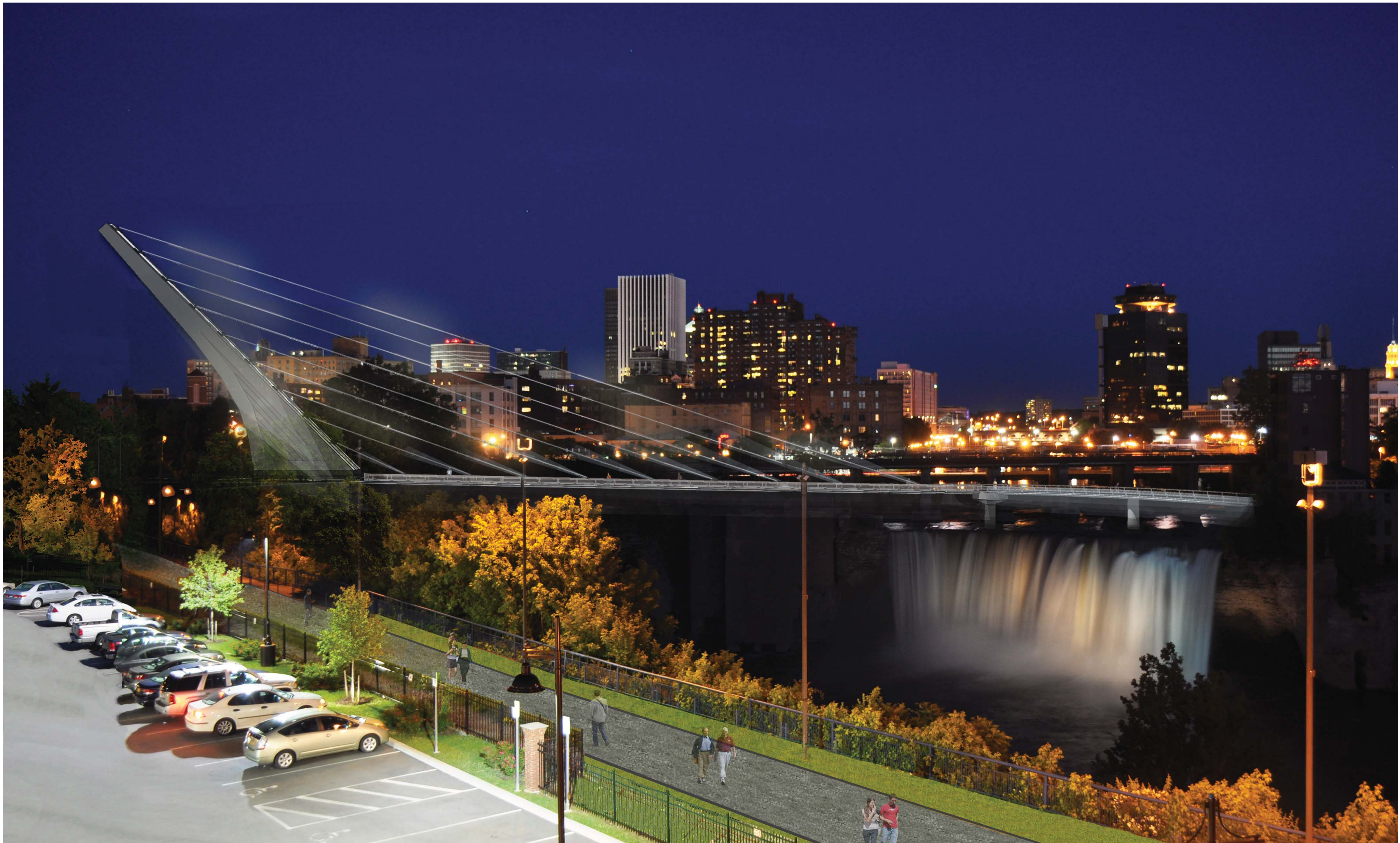
HIGH FALLS PEDESTRIAN ACCESS IMPROVEMENT STUDY BRIDGE CONCEPT 4: CANTILEVER SPAR CABLE STAYED BRIDGE WITH TWO SPAN CURVED GIRDER APPROACH - NIGHTTIME SIMULATION
