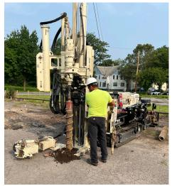
Soil boring and groundwater monitoring well installation to characterize subsurface and collect samples for laboratory analysis.
