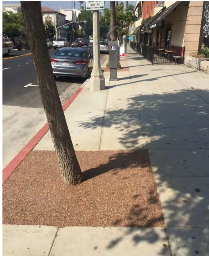
Tree Pit with Porous Pavement
