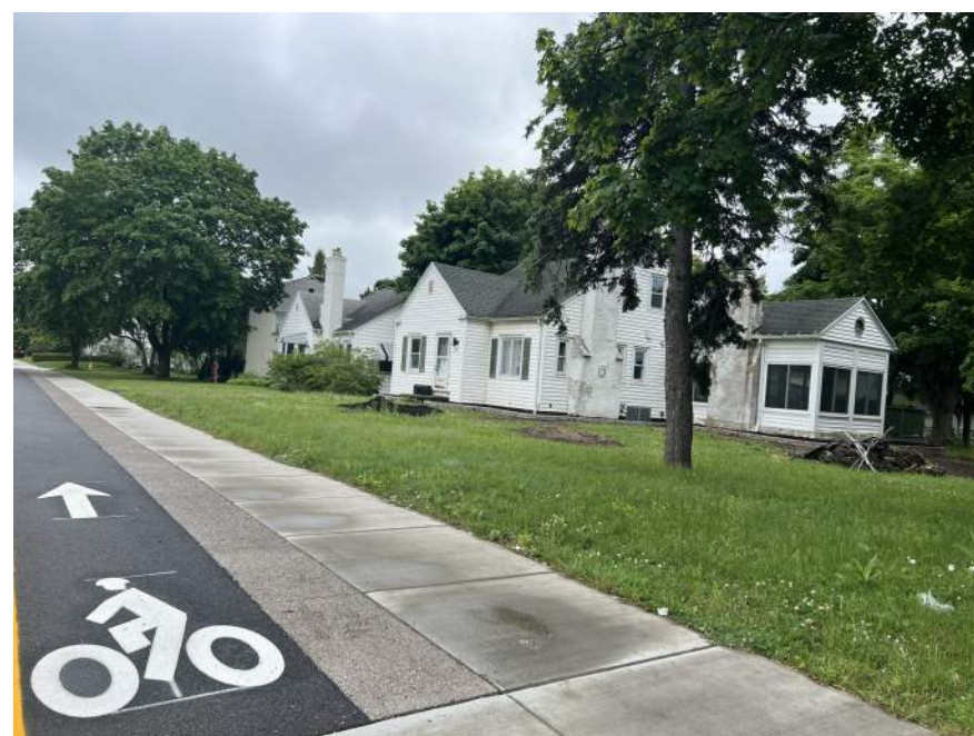
Elevated cycle track on Elmwood Ave with 2' wide exposed aggregate concrete buffer strip and 5' wide concrete sidewalk Similar to one-way cycle track proposed throughout the project
