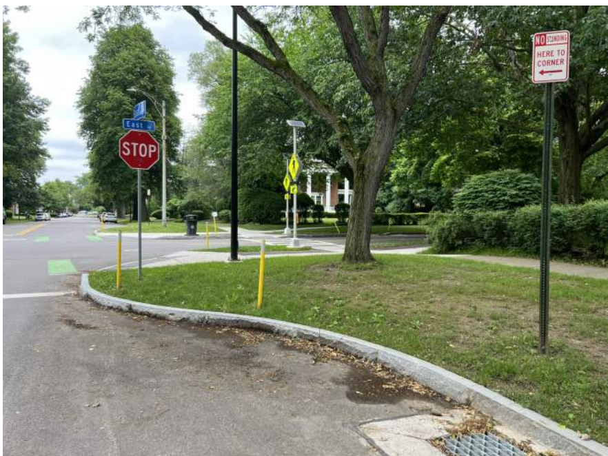
Recessed parking lane on East Blvd at East Ave Similar to recessed parking lane proposed on Genesee St Extension between Silver St and Brown St
