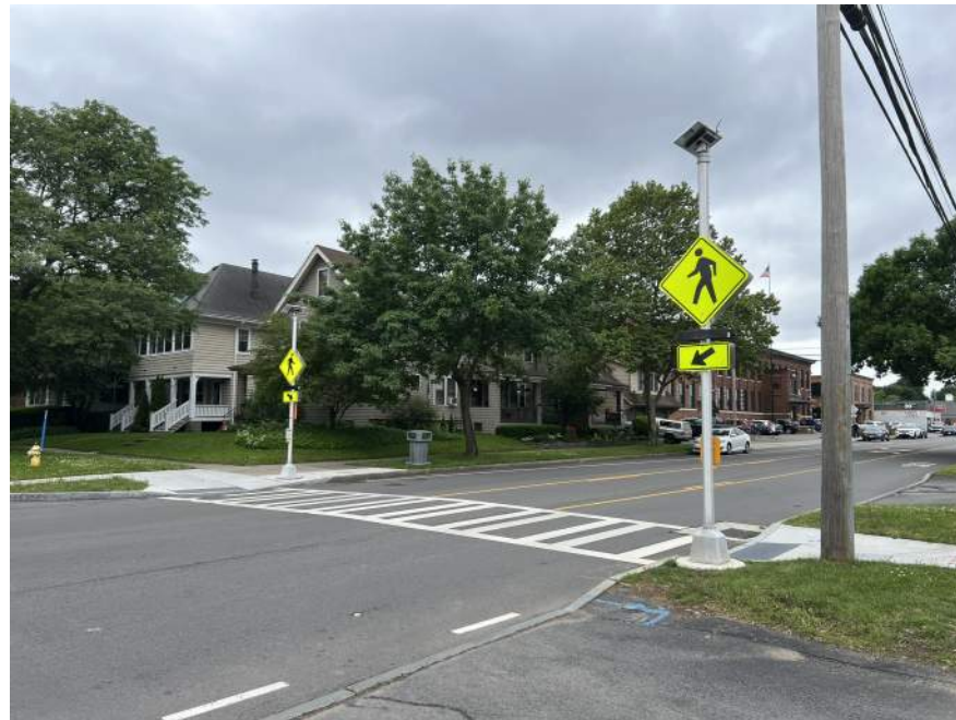
Midblock crossing at University Ave/East Blvd Similar to midblock crossing under consideration at Brown St/Essex St
