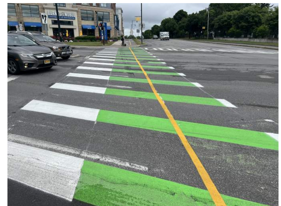
Combined pedestrian/cyclist crosswalk at Mt. Hope Ave/Elmwood Ave Similar to combined crosswalks proposed at W Main/Chili/West and W Main/Genesee, and Genesee Ext./Brown
