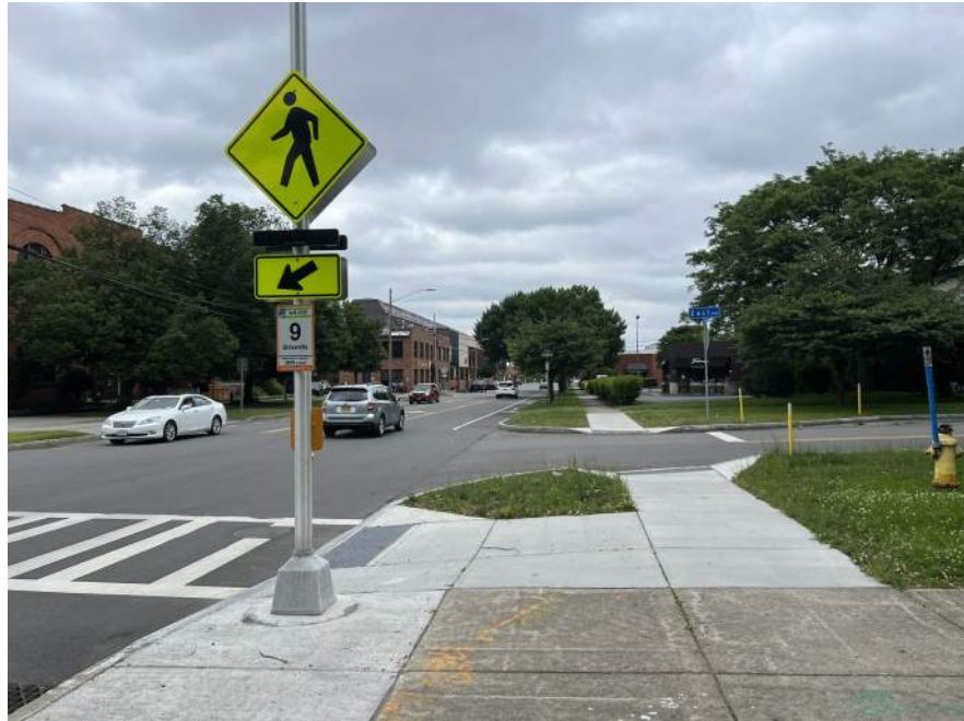
Curb bump out at University Ave/East Blvd Similar to curb bump out proposed at Brown St/Essex St
