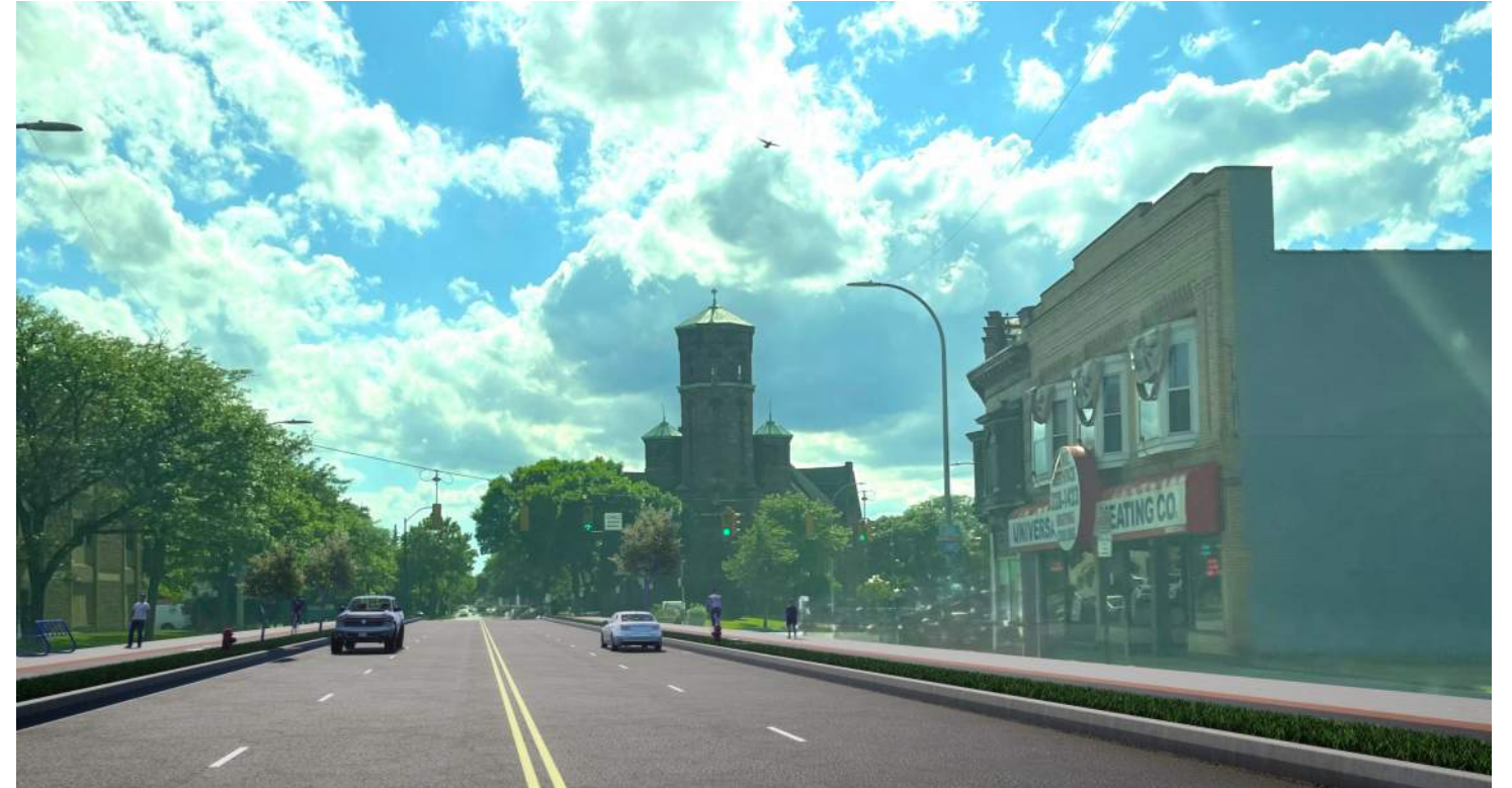
W Main St. facing west towards Chili Ave. at West Ave.
