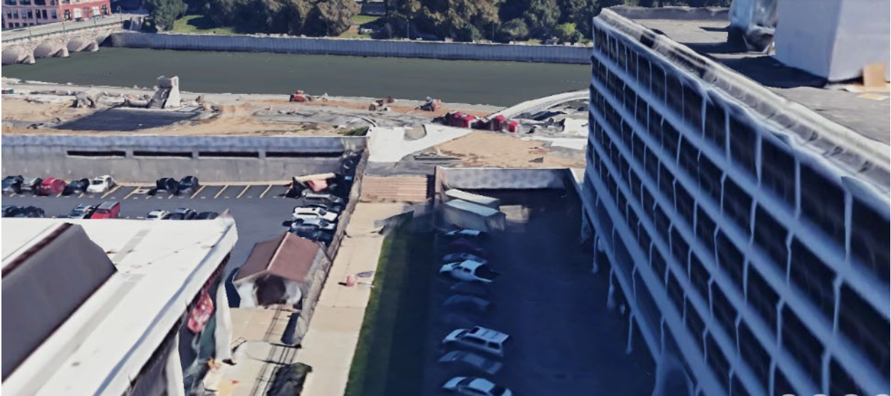
State Street Connection looking east toward Austin Steward Plaza. Genesee Crossroads Park in distance across Genesee River. Federal Building to left and Holiday Inn to right.
