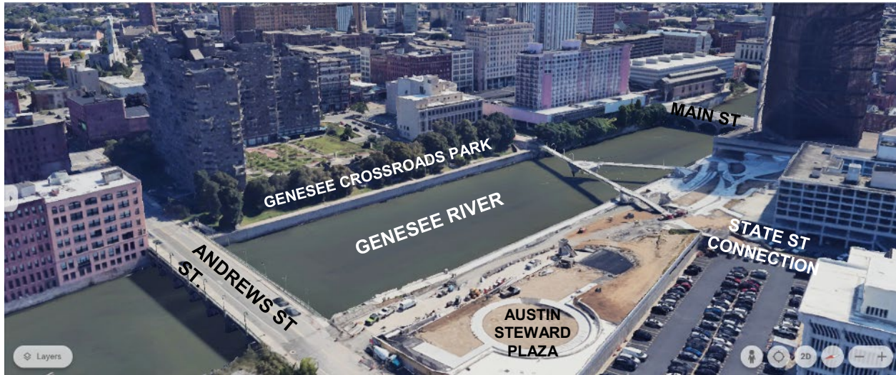
Aerial view of project area looking southeast.
