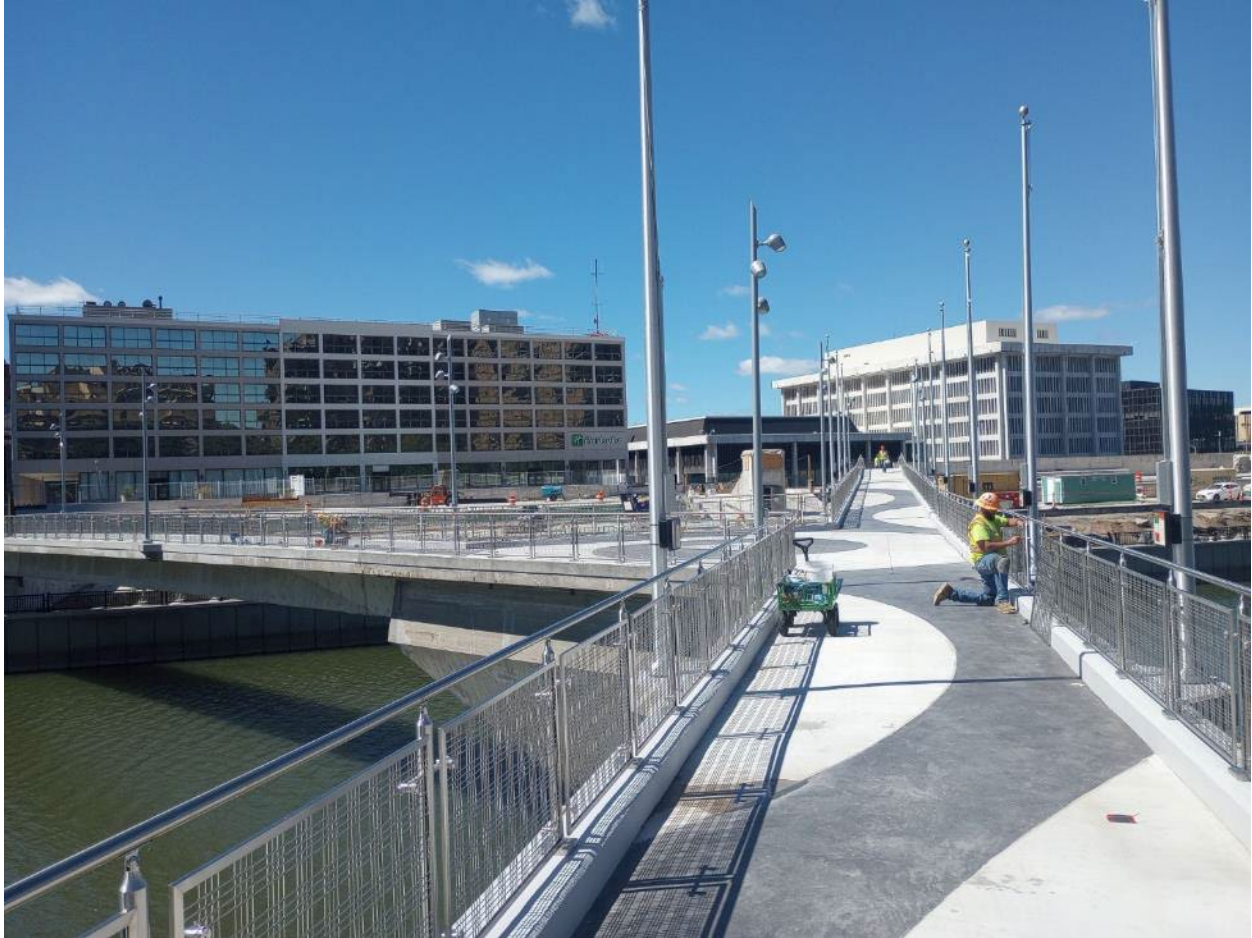
Looking northwest toward the center point of the Sister Cities Bridge.
