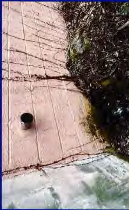
building drainage onto site
