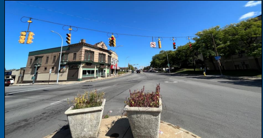
View looking northeast from Chili Ave/West Ave (W. Main St/Chili Ave/West Ave/York St Intersection)
