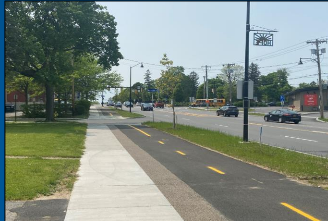
Two-Way Cycle Track Elmwood Avenue
