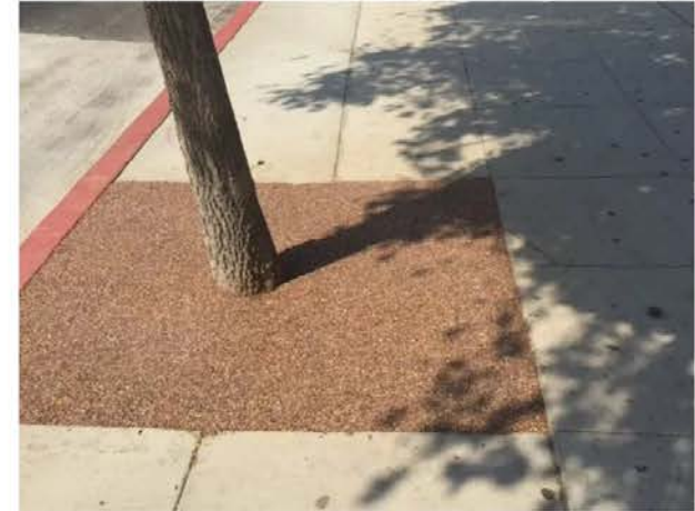
Tree Pit with Porous Pavement
