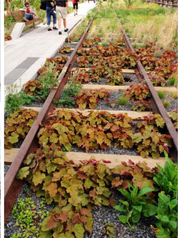
Opportunities to integrate native plantings into historic railroad structures highlights a merging of nature and history
