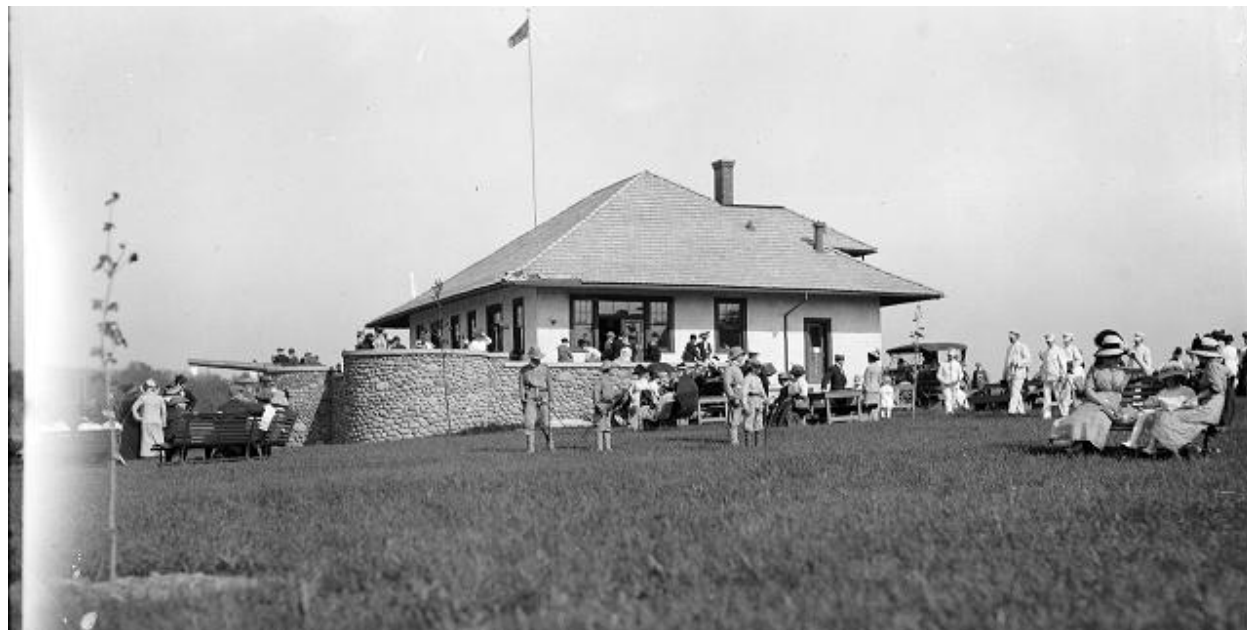
The Refectory was used by guests as a point to get refreshments. The patio foundation still stands today as “White Lady’s Castle.”
