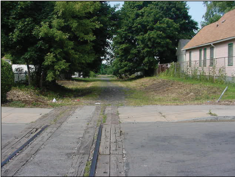
Rochester Running Track intersection with Scrantom Street
