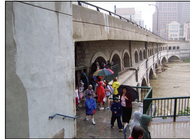
Visitors peek into the old Erie Canal Aqueduct under Broad Street
