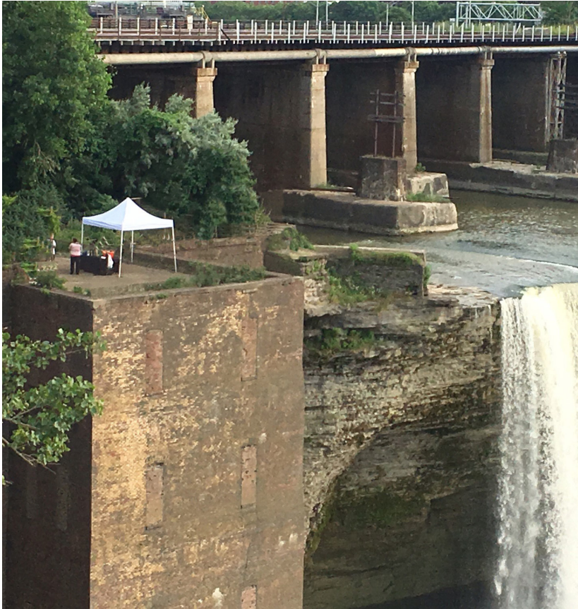
VIEW OF FORMER RG&E HYDROSTATION #4 | LOOKING SOUTH
