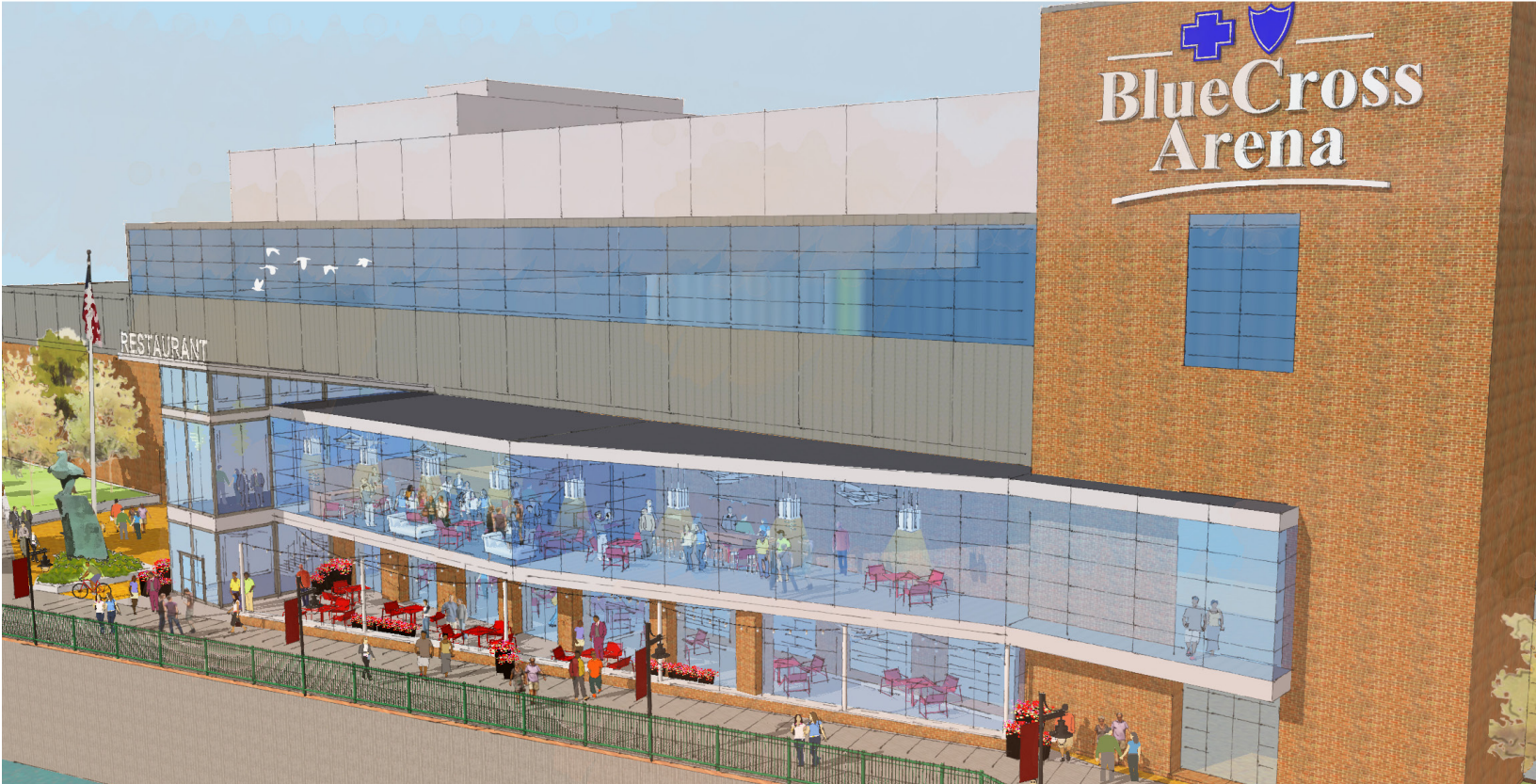
BLUE CROSS ARENA | RIVER SIDE
