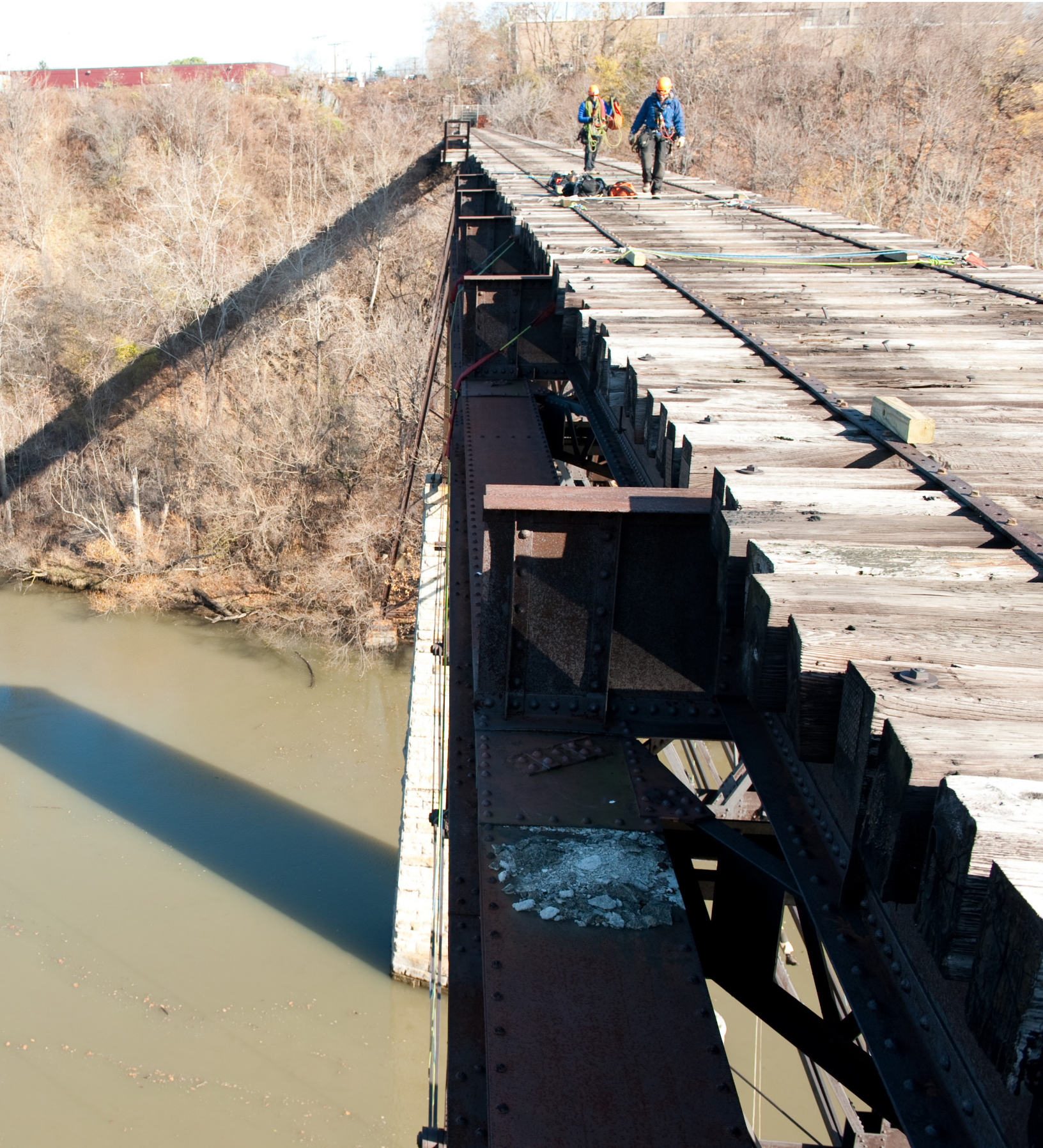
RUNNING TRACK BRIDGE | LOOKING EAST
