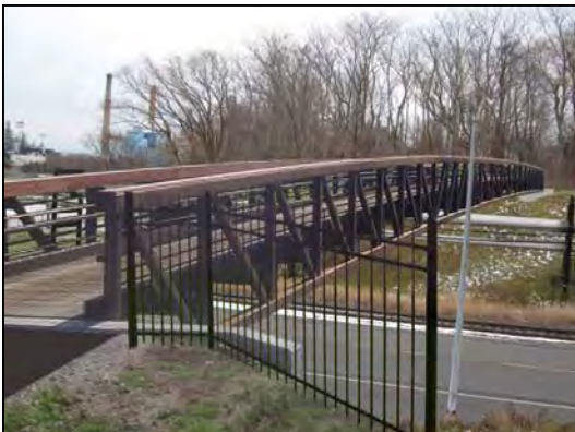
Figure 5-1. Photo rendering showing a conceptual pedestrian bridge over Kodak Park Avenue along the former Eric Canal corridor.
