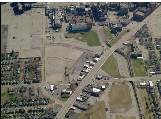
EBP’s vast parking lots and redevelopment sites provide opportunities for locating a multi-use trail.
