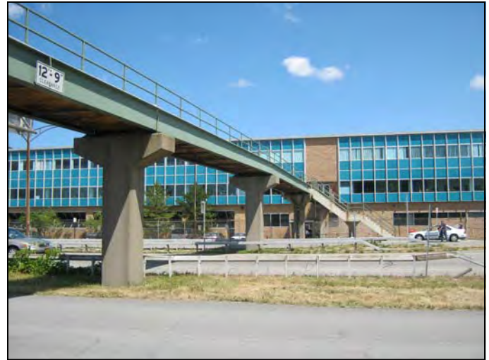
Pedestrian bridge over Mt. Read Boulevard connecting to Building 205 in EBP.
