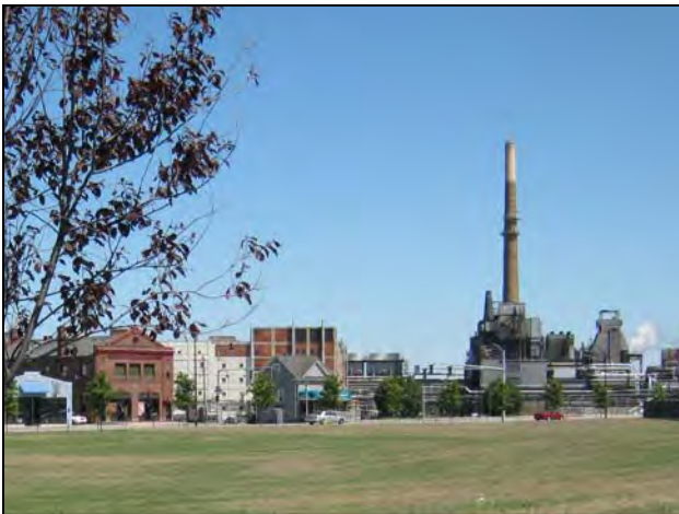
Commercial uses on West Ridge Road in the shadow of Eastman Business Park.
