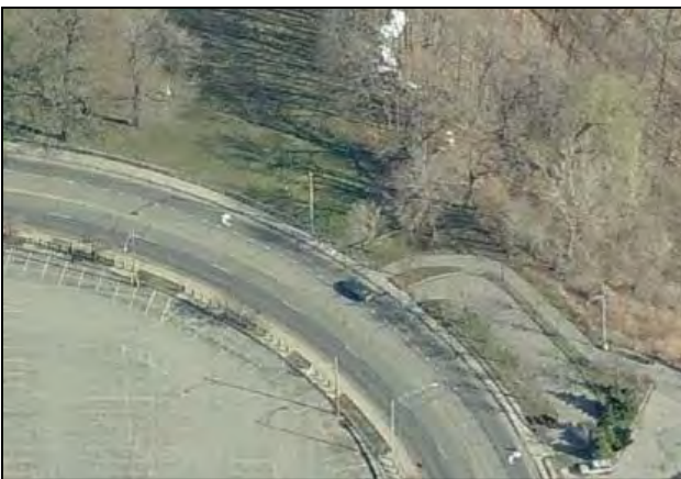
The parking lot adjacent to King's Landing Cemetery is a potential location for a trail head with kiosks, benches, restrooms, and other amenities.
