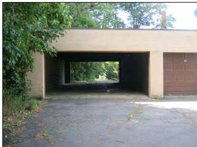
The vertical clearance of the garage behind St. Bernard's exceeds the minimum required by state and national guidelines.
