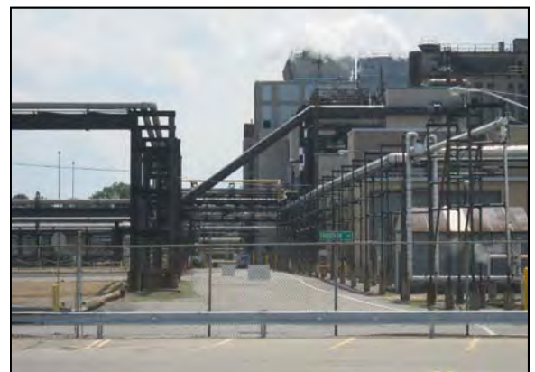
Industrial infrastructure in Eastman Business Park.
