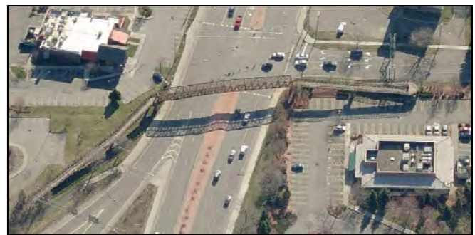
Southern terminus of the Route 390 Trail, where a pedestrian bridge carries trail users over West Ridge Road.
