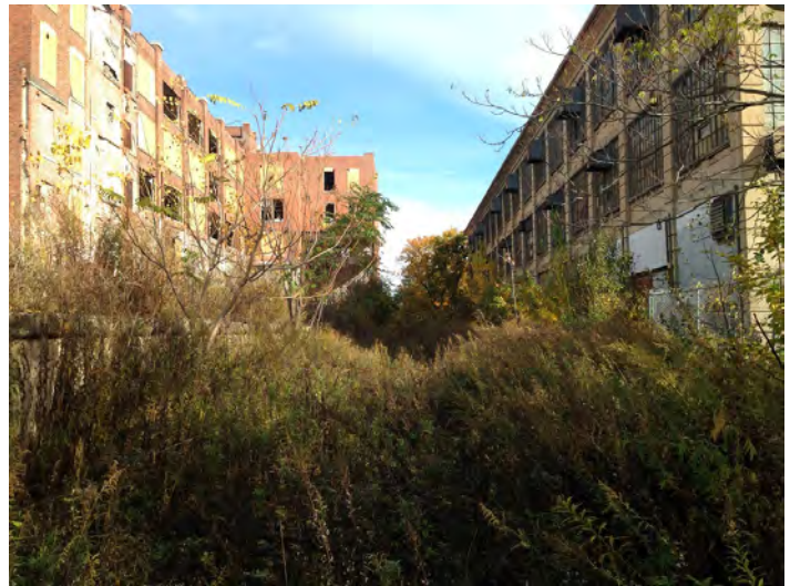
Looking east towards Orchard Street.
