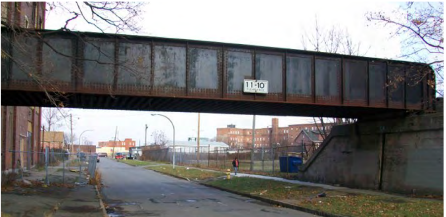
Orchard Street Bridge, looking north.
