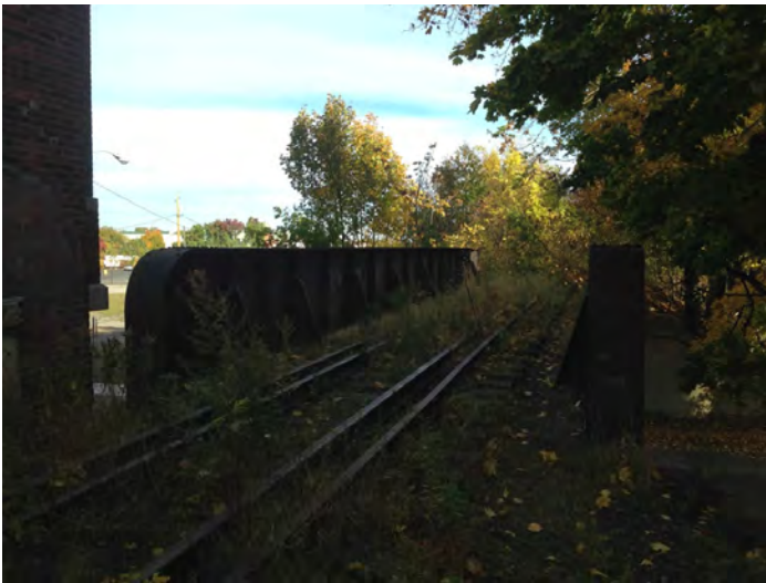
Orchard Street railroad bridge looking east.
