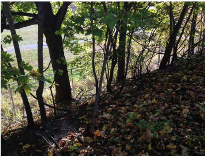
Steep embankment to the south of the corridor and adjacent to the Sahlen's Stadium overflow parking lot.
