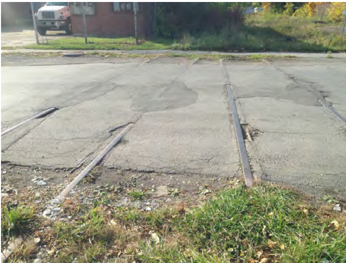
Three sets of tracks at Whitney Street intersection looking west.
