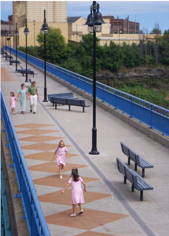
Pont de Rennes Pedestrian Bridge
