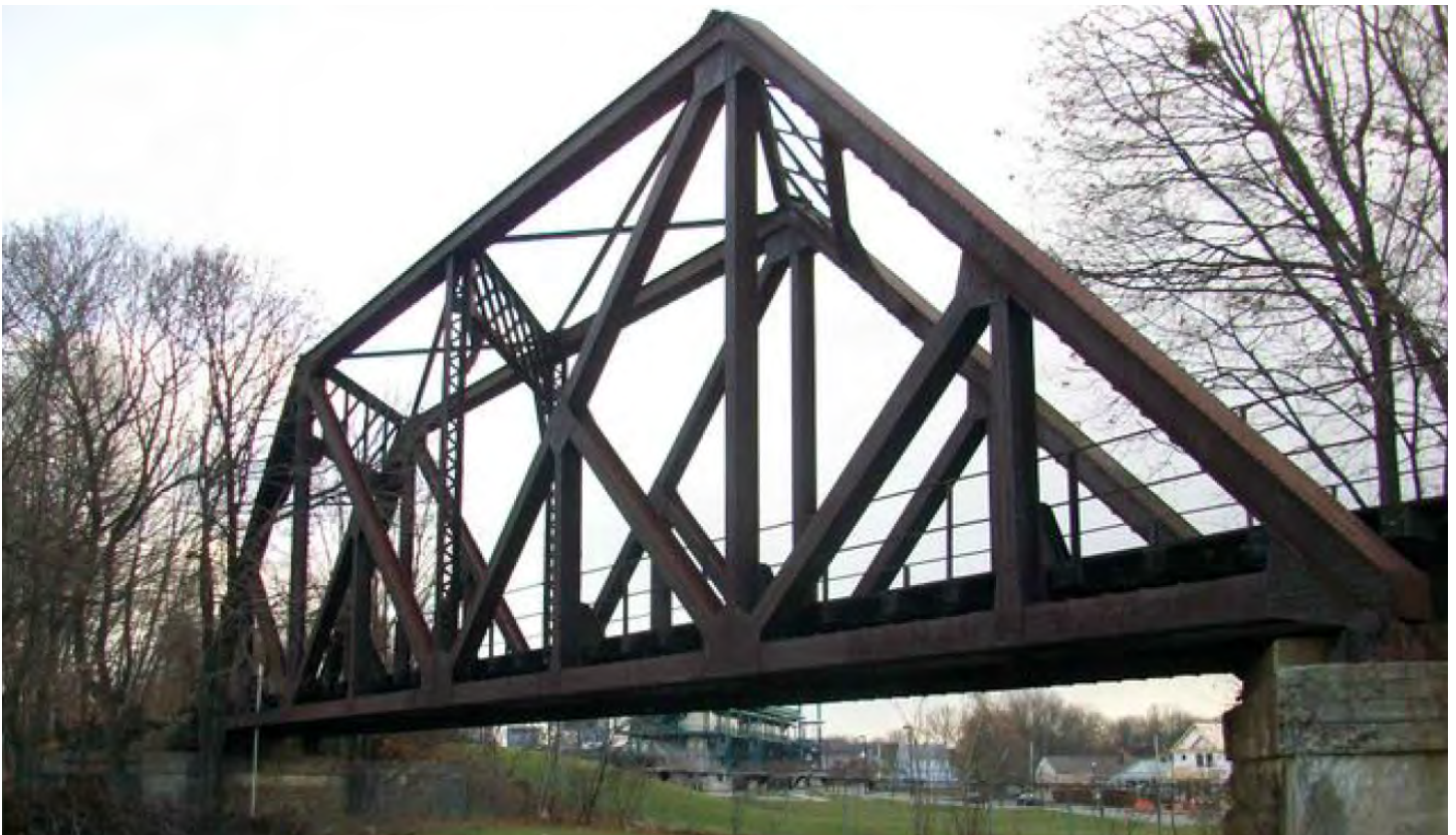
Bridge over former Erie Canal Bed - Span 5, looking south.
