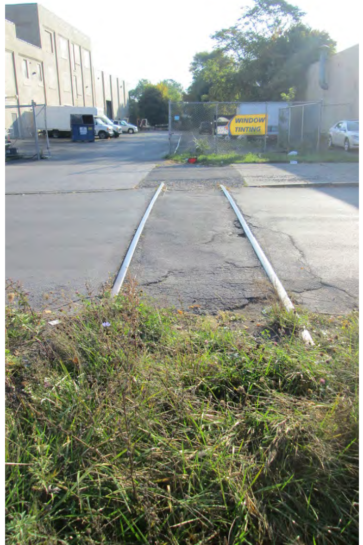
Murray Street intersection looking east.
