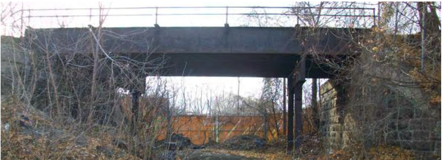
Moore Street Bridge, looking north.
