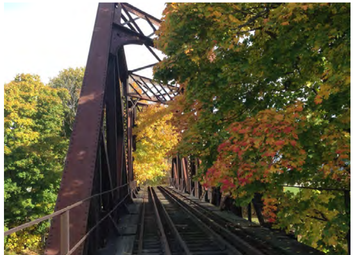
Railroad bridge over former Erie Canal looking east.
