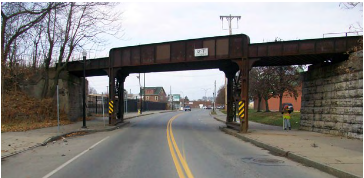
Broad Street Bridge - Spans 1-3, looking north.
