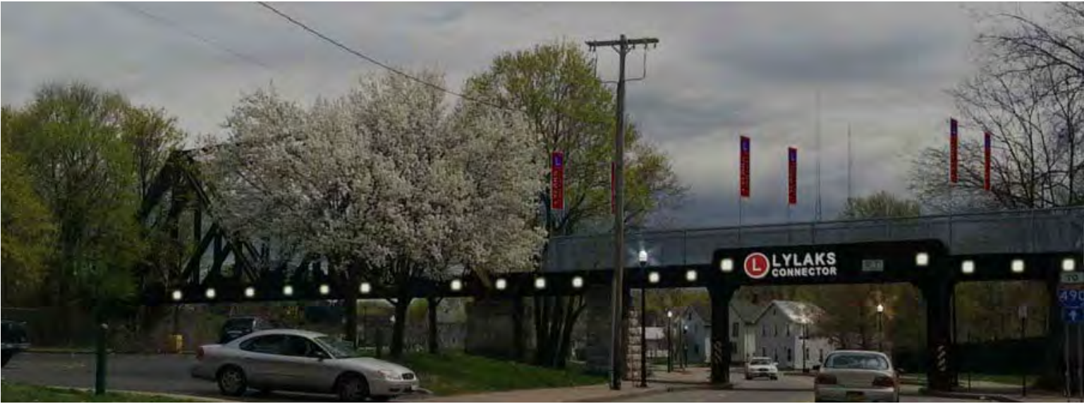
Lighting concept for the Broad Street railroad bridge. Innovative LED or solar light could be potential options for lighting the bridge.
