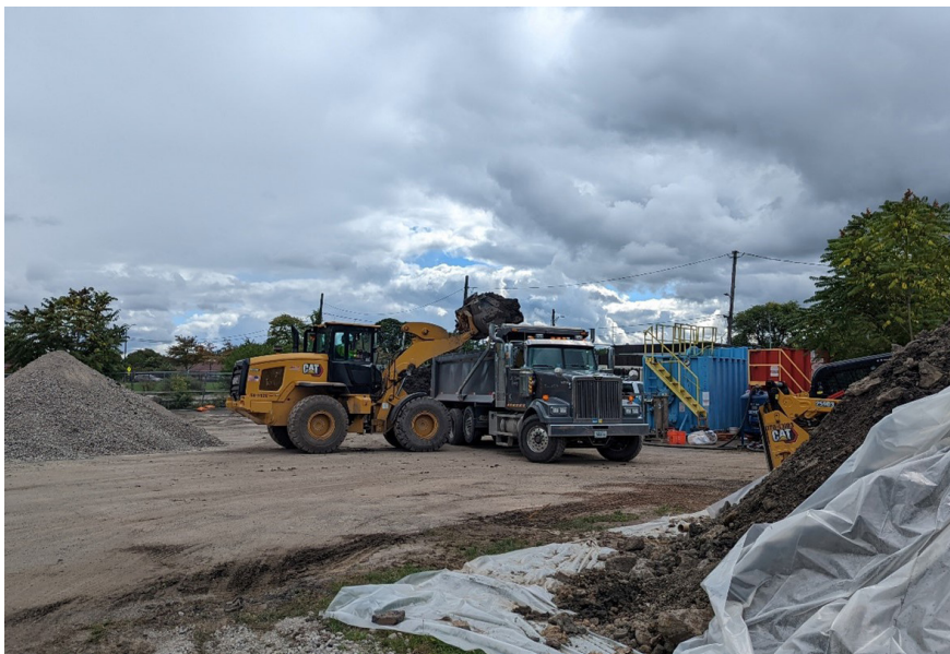
Typical Loadout Activities
