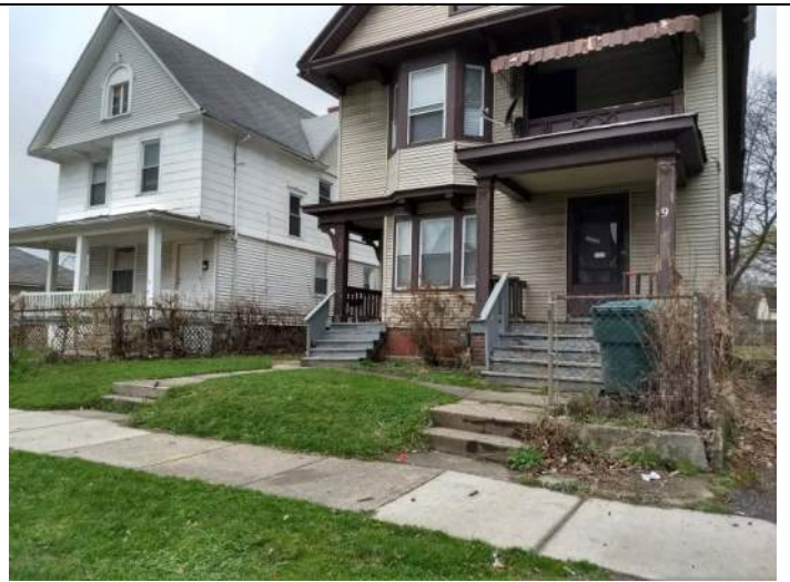
South adjacent properties
