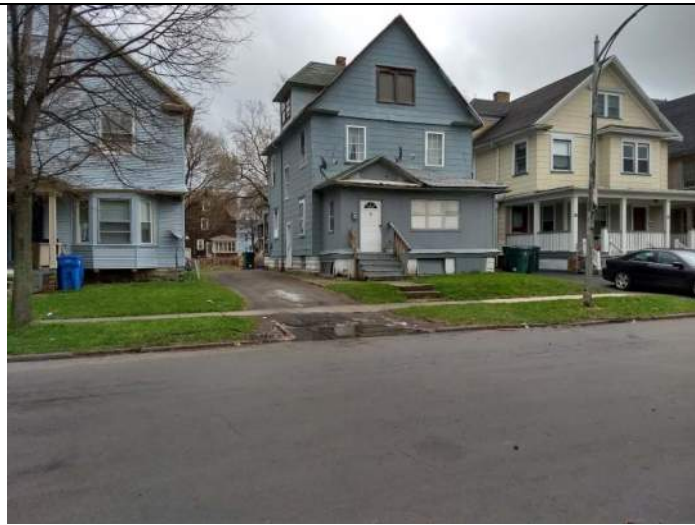
East adjacent properties
