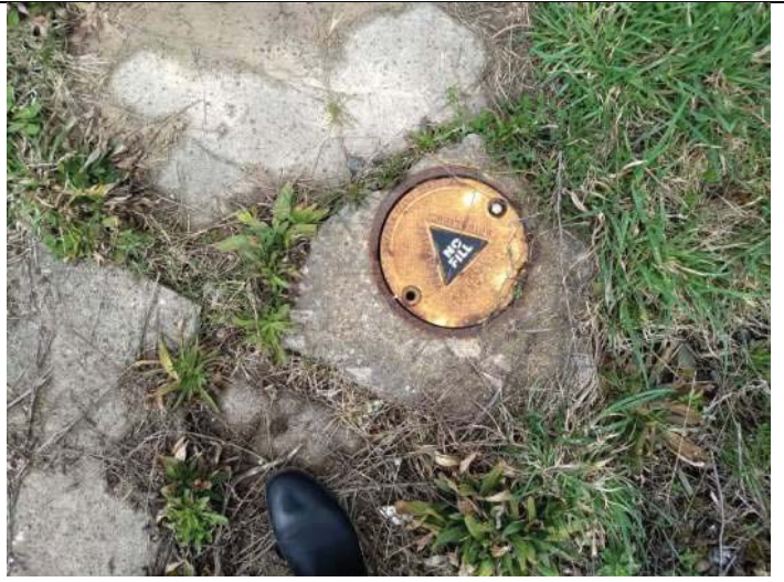
Monitoring well on-Site
