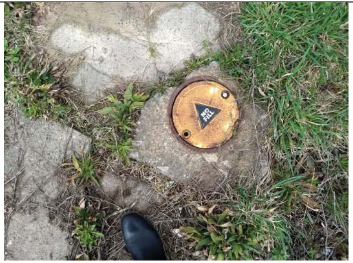
Monitoring well on-Site
