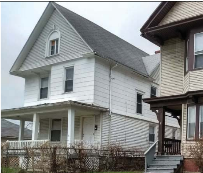
North adjacent property
