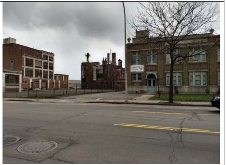
South adjacent property
