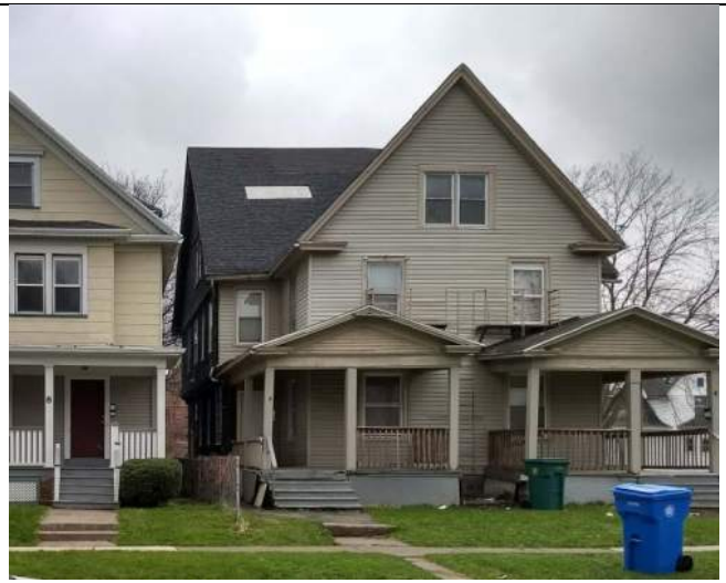
North adjacent property
