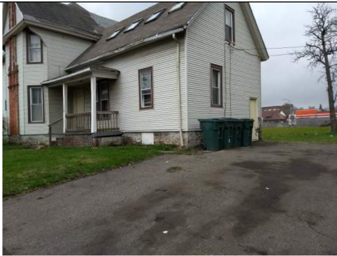
West adjacent property
