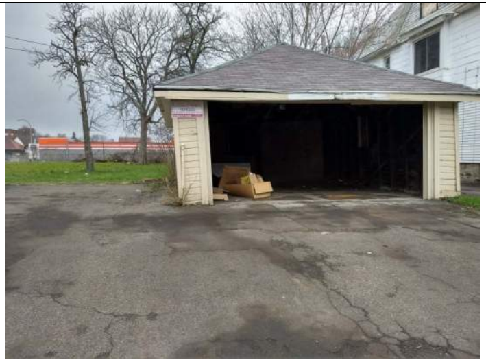
West adjacent property
