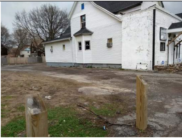
Southeast adjacent property
