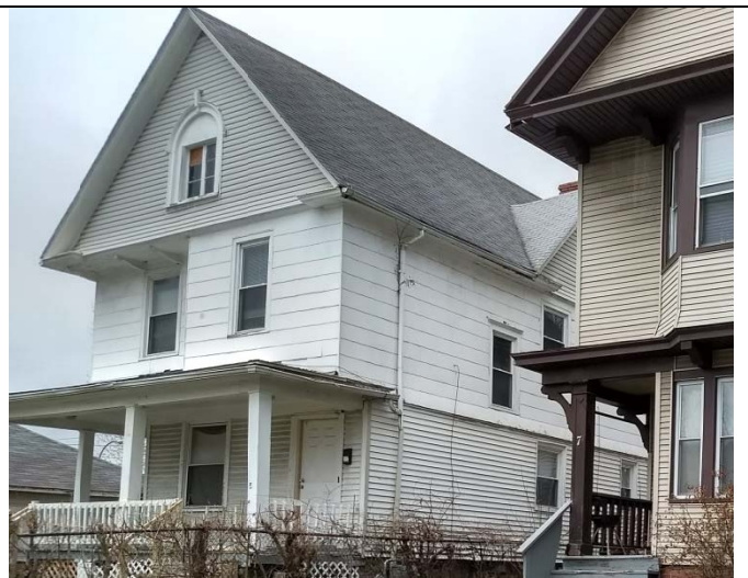
South adjacent property
