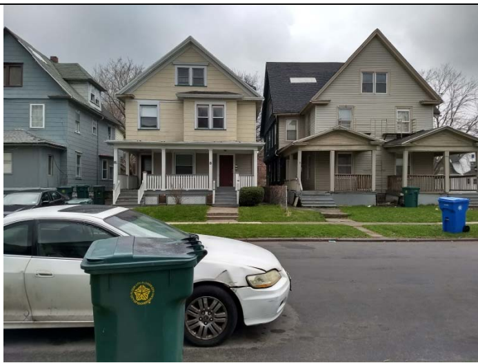
East adjacent properties
