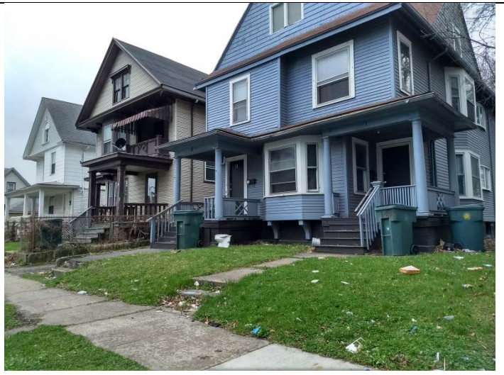
North adjacent property
