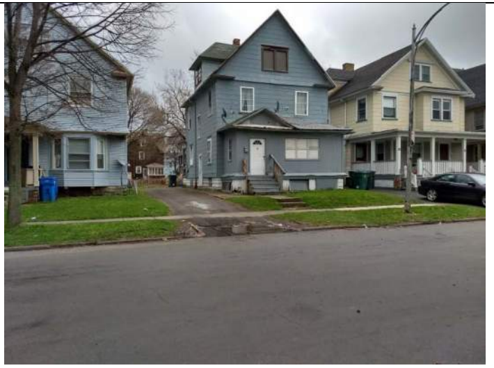
North adjacent property
