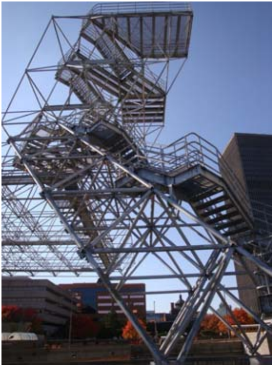
Manhattan Square Park, scaffold-type structure with platforms above plaza, 2009.
