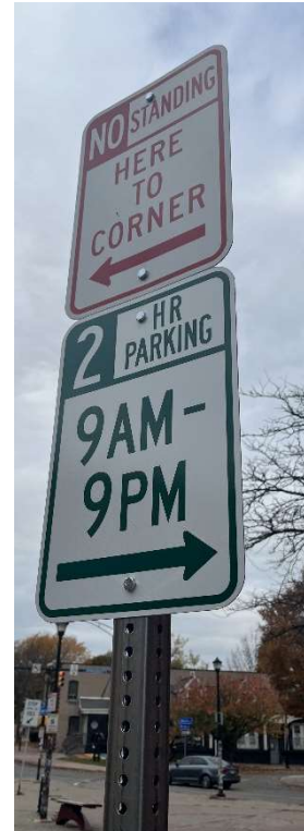
Photo Description Post Mounted Sign Good Reflectivity Sign and Post to Remain
