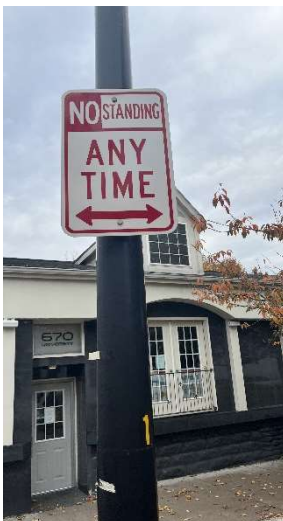
Photo Description Pole Mounted Sign (Band Mounted) Good Reflectivity Signs to Remain
