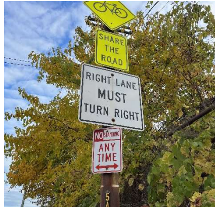
Photo Description Pole Mounted Signs (Band Mounted) Good Reflectivity Signs to Remain
