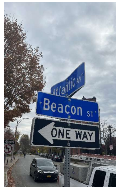
Photo Description Post Mounted Sign Damaged Sign Sign (only) to be Replaced
