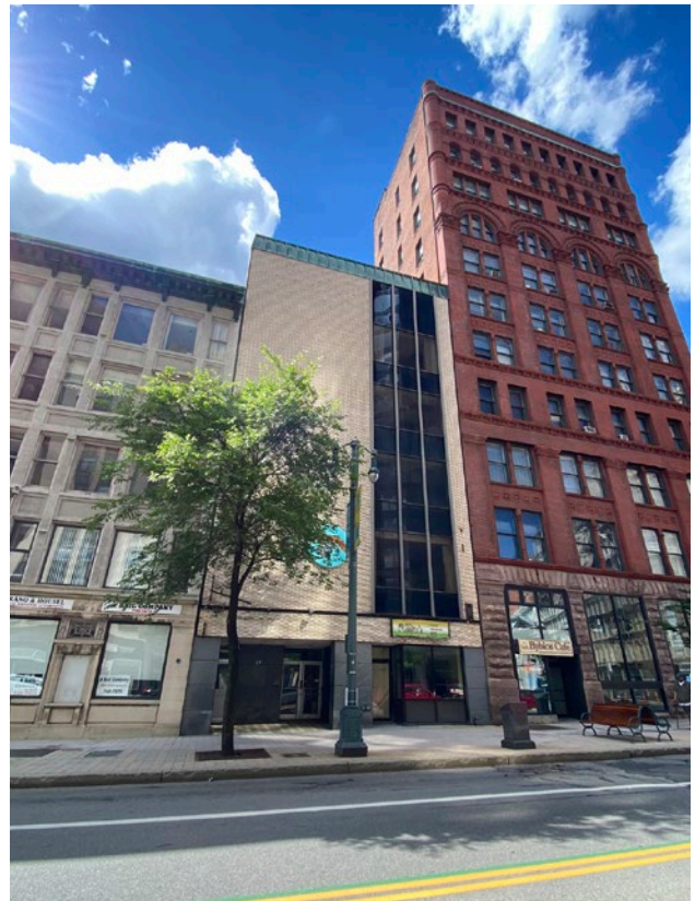
Existing: 17-21 E. Main Street building.
