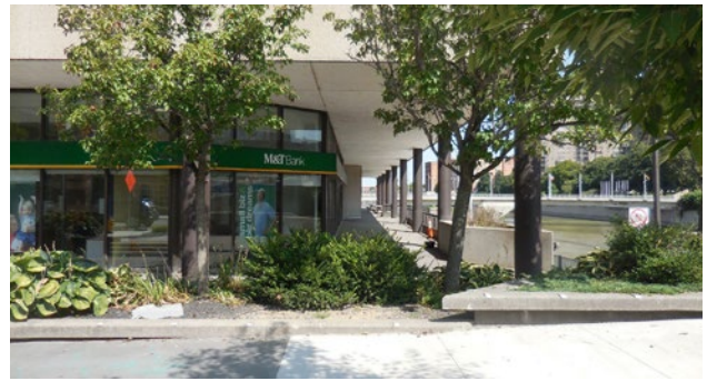
Existing: Unclear connection to plaza, view from Main Street.
