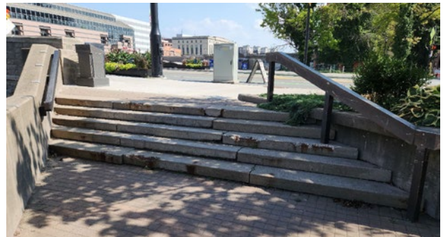
Existing: Staired access from Main Street, looking south.
