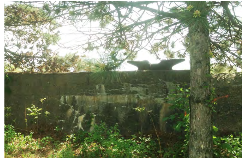
AN OBSTRUCTED VIEW OF THE RIVER FROM THE RIVERWAY TRAIL. NOTE THIS HISTORIC CLEAT ATOP THE WALL.
