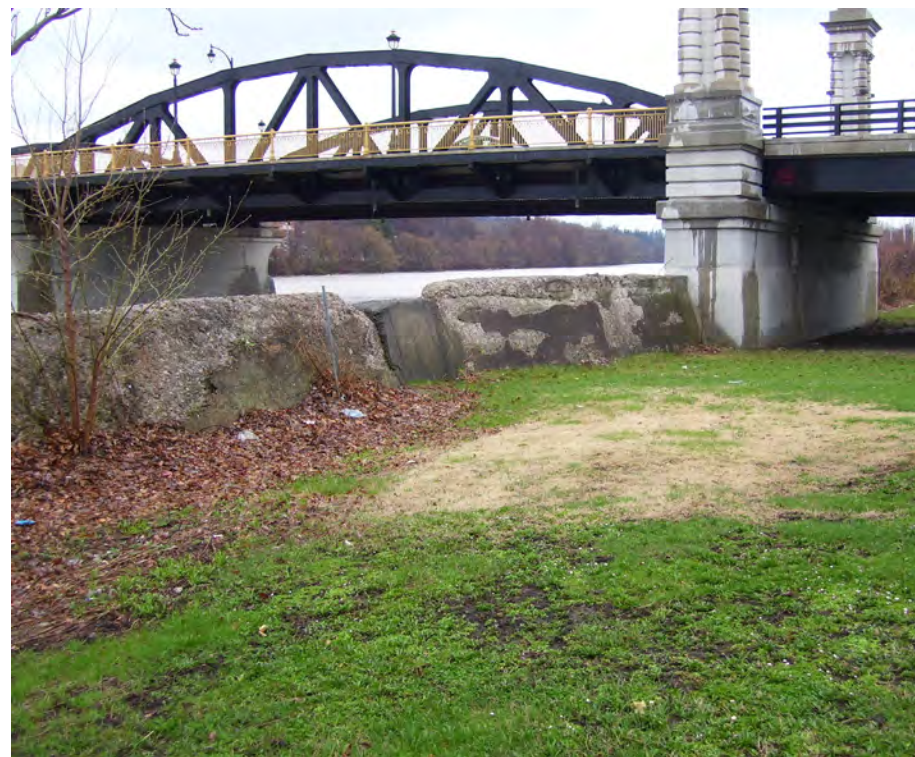
VIEW OF WALL LOOKING SOUTH TOWARDS FORD STREET BRIDGE
