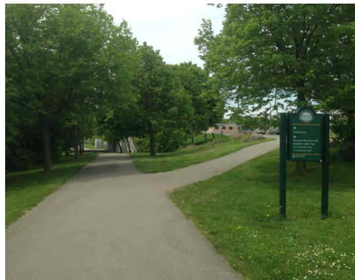
GENESEE RIVERWAY TRAIL LOOKING SOUTH TOWARDS FORD STREET BRIDGE
