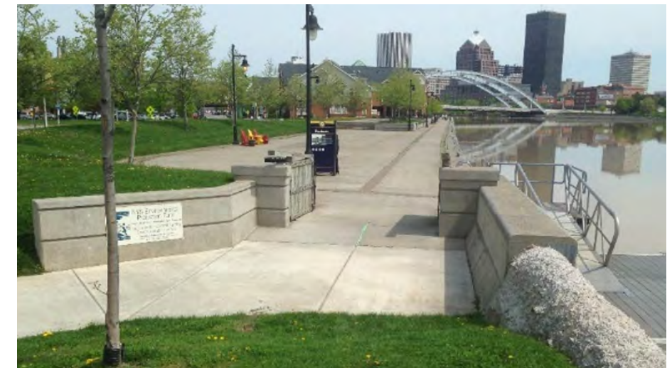
THE RIVERWAY TRAIL LOOKING NORTH TOWARDS CORN HILL LANDING, SHOWING EXISTING FLOOD GATES AND THE TRANSITION FROM OLD TO NEW SECTIONS OF THE RIVER WALL
