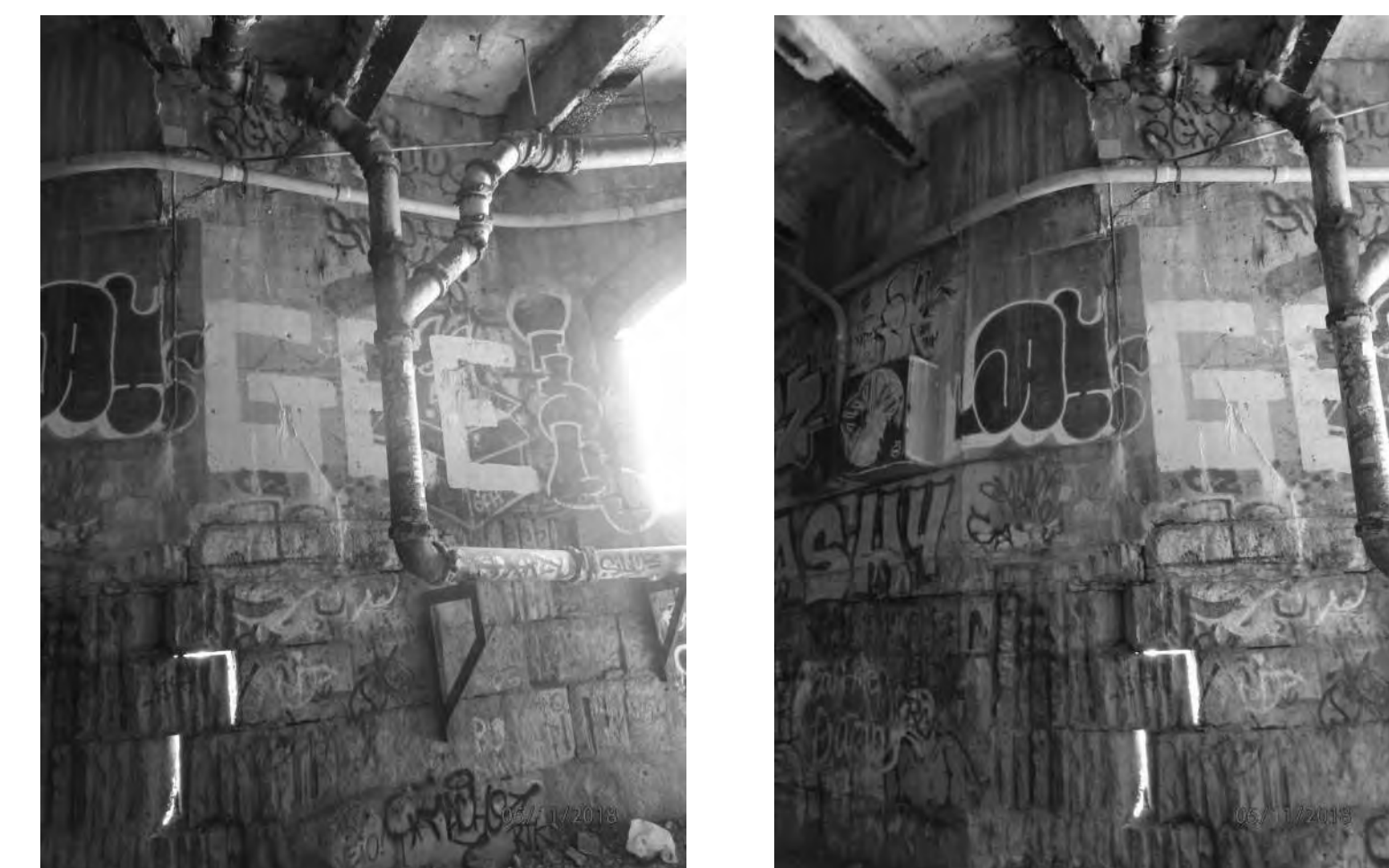
PHOTO LOCATION A - WALL REPAIR - EXISTING CONDITIONS
