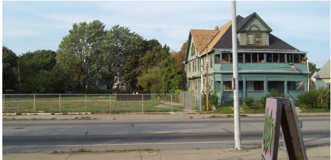
1200 & 1214 East Main Street are challenges the community can overcome.
