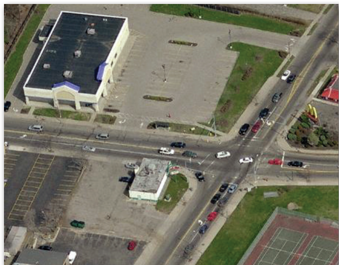
Existing Gateway Condition
