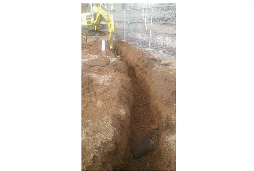
Excavation for the SVE trench along the 1214/1216 residential home
