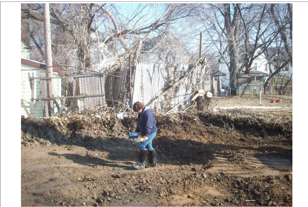
Air monitoring near residential property line
