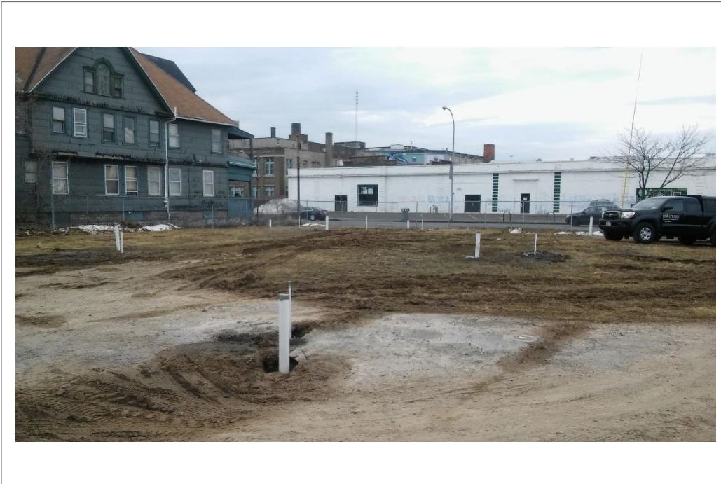
VEGE Extraction Wells and O2 injection points
