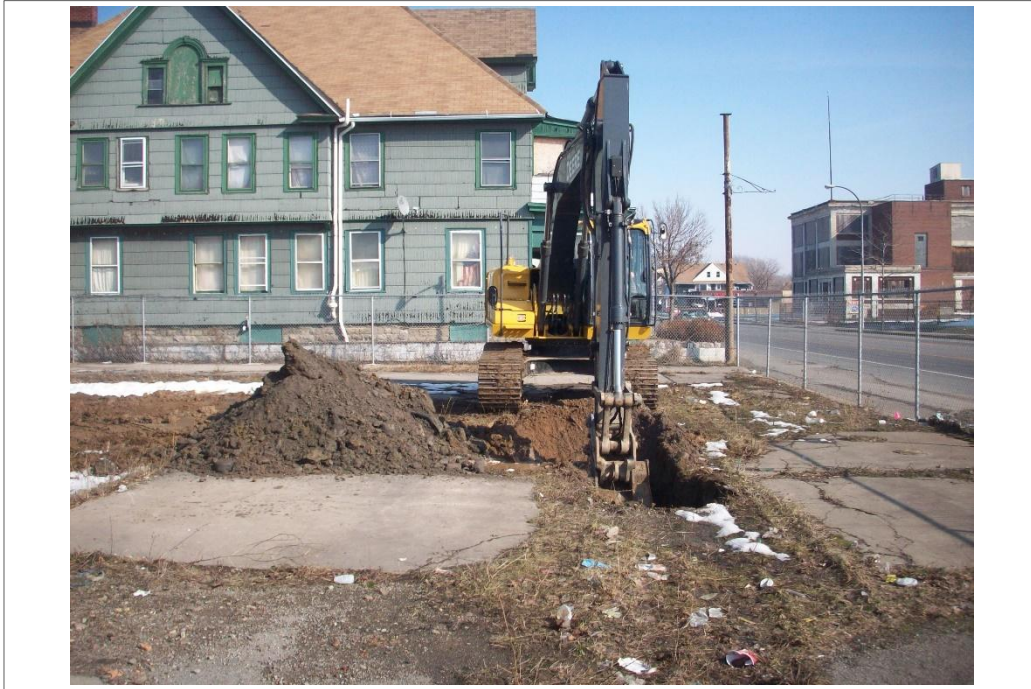
Excavation of Area 3 – March 2010
