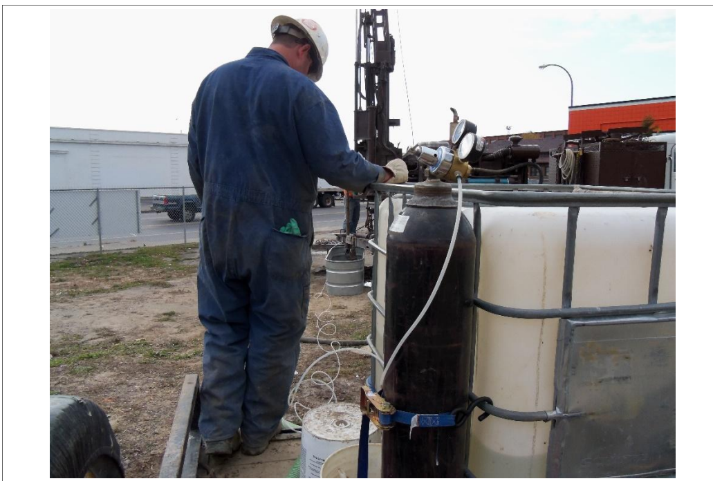
Nitrogen supply line to inflate packer in bedrock ISCO injection zone
