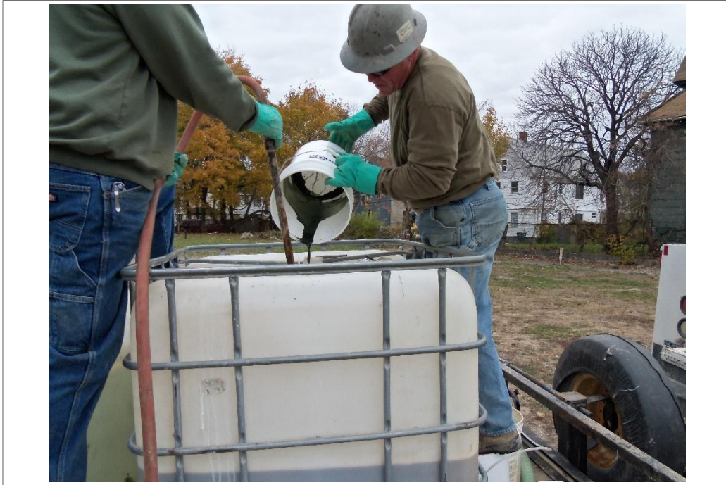
Batch mix of RegenOx for ISCO injections
