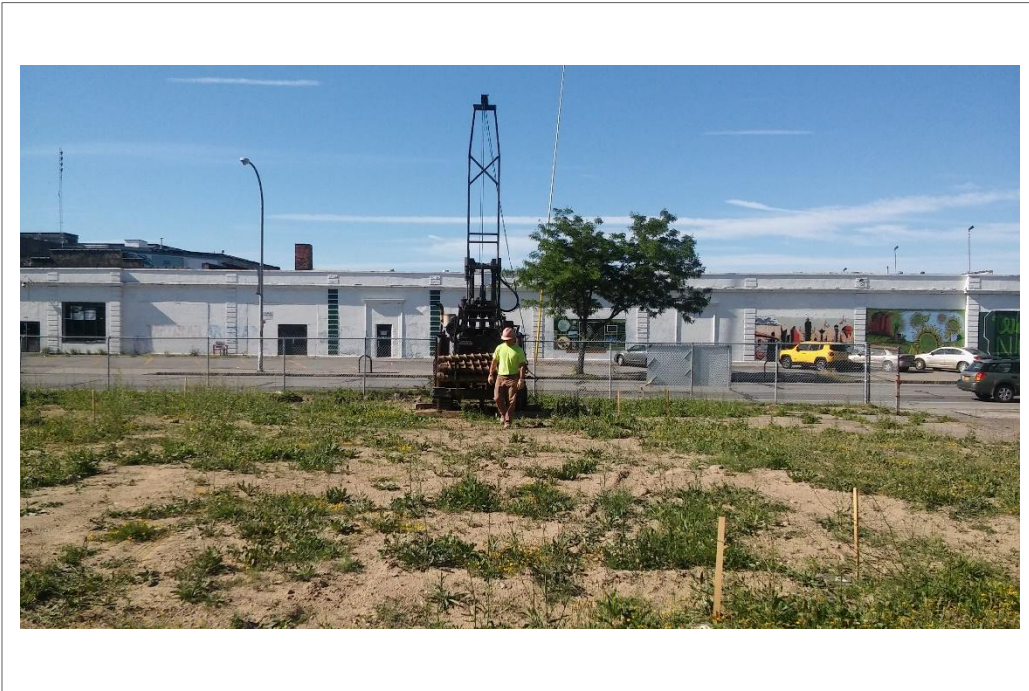
Installation of Oxygen Injection points
