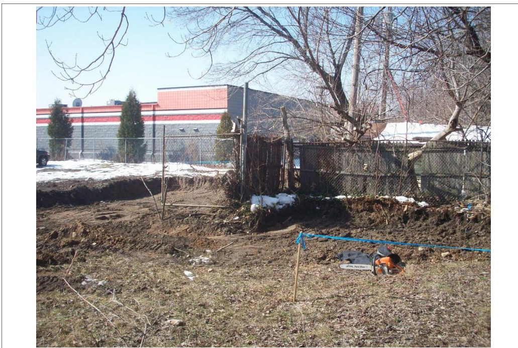
Excavation at Area 1B – March 2010
