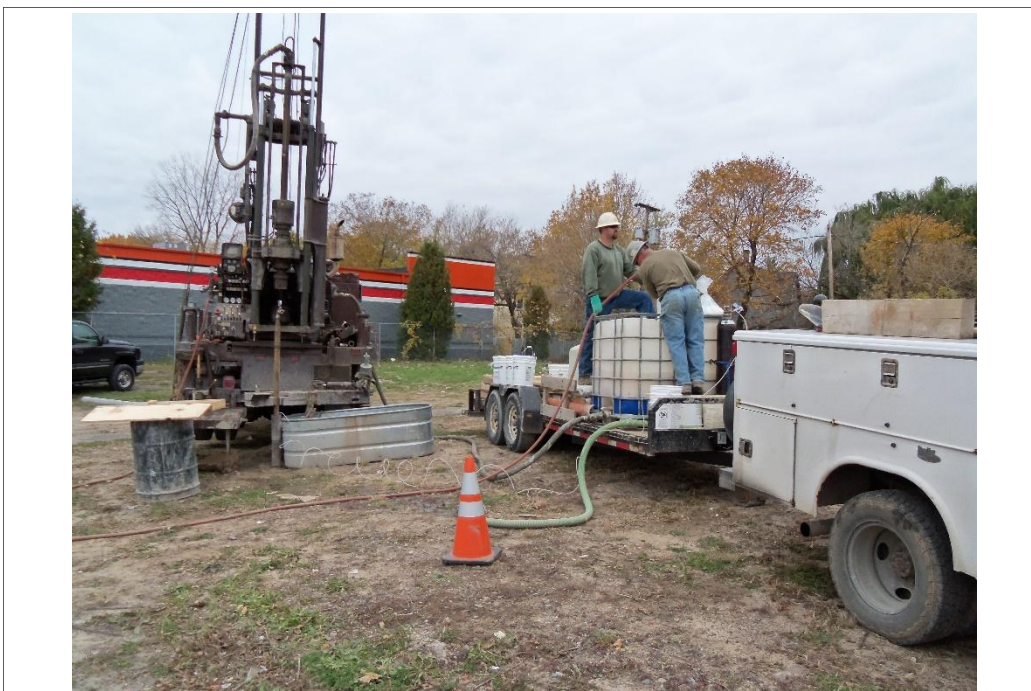
Mixing RegenOx slurry at Treatment Area 1 – ISCO December 2011
