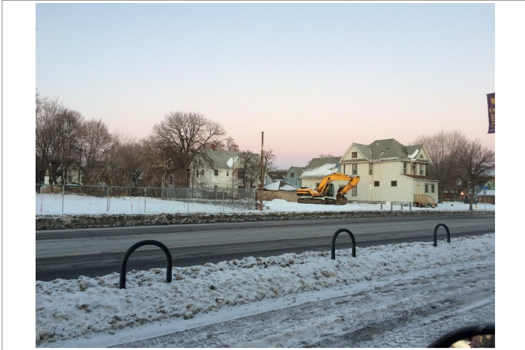
View of Site and demolished 1214/1216 E. Main Street - December 2016
