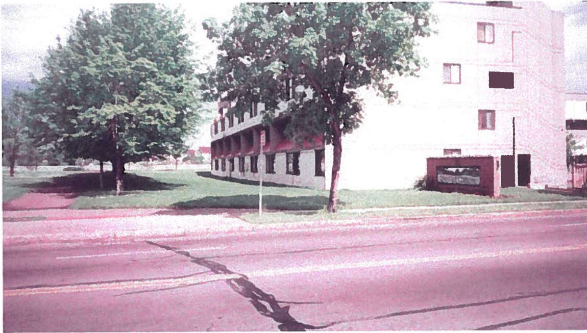
View of the low-rise apartment buildings looking to the west.
