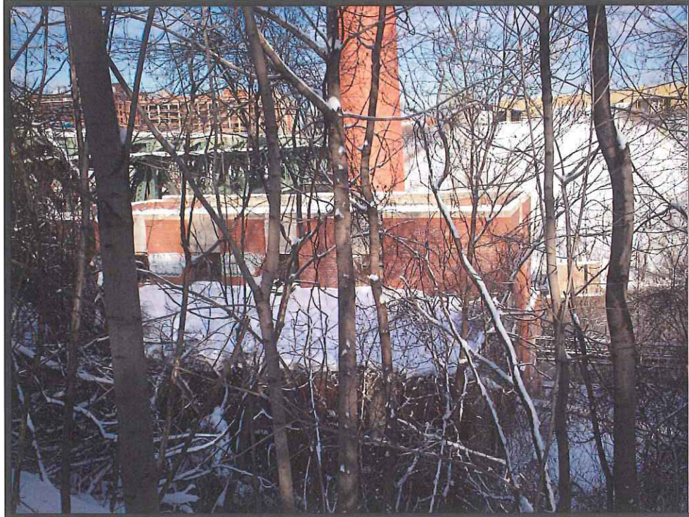
View of the former City of Rochester Incinerator/Garbage Reduction Plant located adjacent to the east of the Site.
