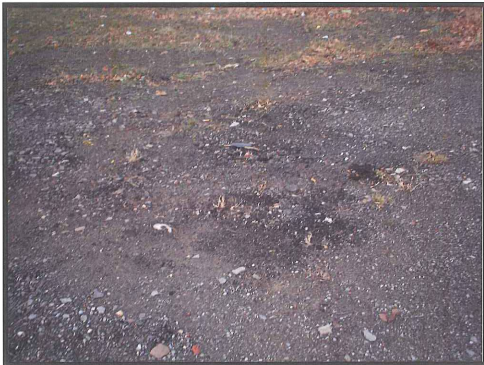
View of surface soil at the Site containing cinders and scrap metal as well as brick, concrete, and coal fragments.
