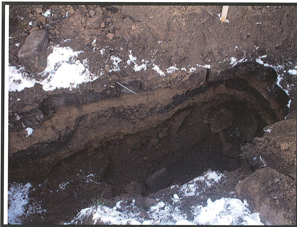
View of the TP-111 featuring pavers of former roadway underlain by coarse sand, fill materials layer, and native soil
