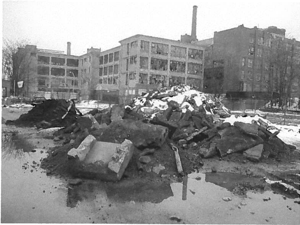
Debris located on 350 Orchard Street parcel
