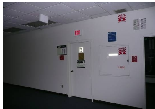
6 th Floor of Seneca Building
