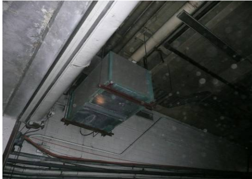
Underground service tunnel
