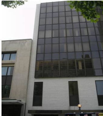
East view of Seneca Building
