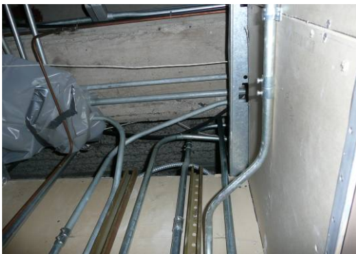
6 th Floor of Seneca Building
