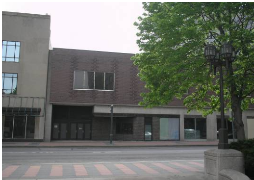
East view of vacant building south of B. Forman Building
