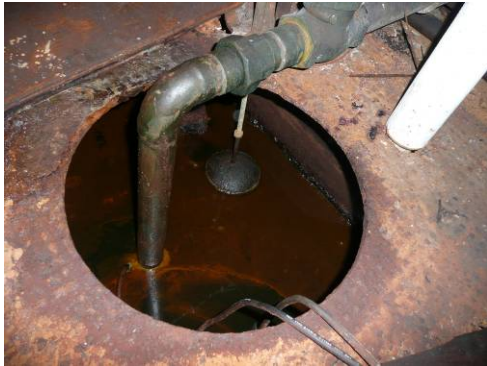
Sump in sub-basement of McCurdy's Building
