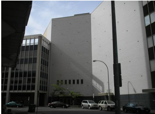
Southwest view of McCurdy's and Euclid Buildings
