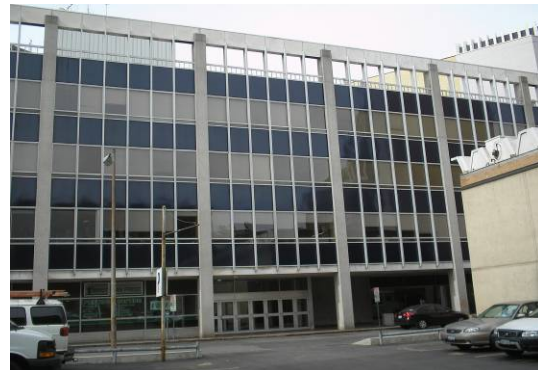
Southwest view of Euclid Building
