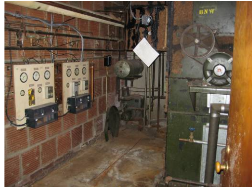
Mechanical room in basement
