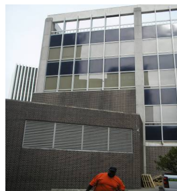
Southwest view of Euclid Building
