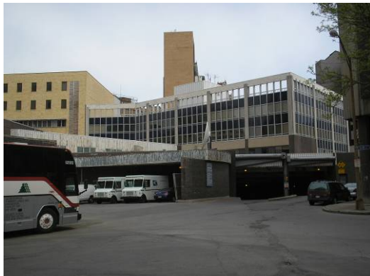
Northeast view of Euclid Building and entrance to underground service tunnel near Atlas and Elm Street
