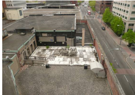
Roof of B. Forman Building
