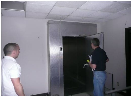
Refrigerator room for computer at Seneca Building
