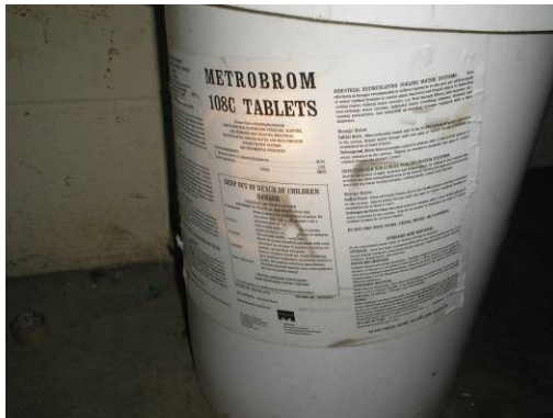
Treatment for cooling water system
