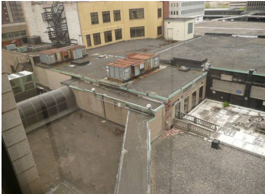
Roof of B. Forman Building
