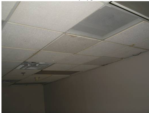
Fluorescent light fixtures 6 th floor
