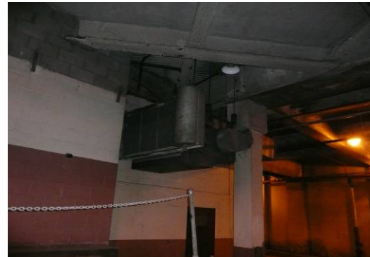
Underground service tunnel door opener
