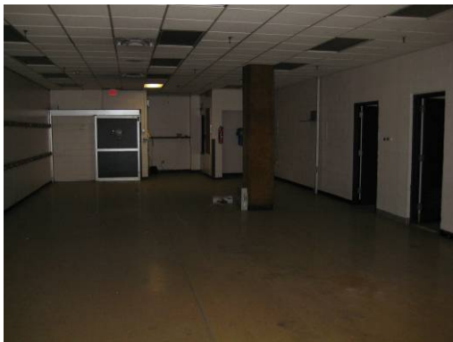
Southwest end of Room 7 in basement
