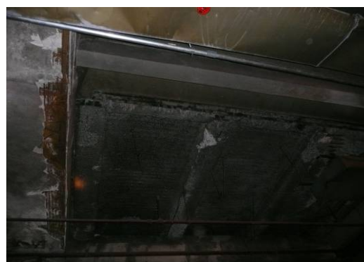
Spray-on ceiling at underground service tunnel near McCurdy's Building
