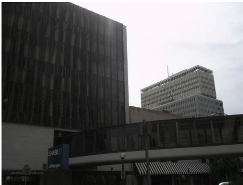
Southeast view of Seneca Building
