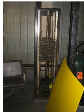
Equipment on roof
