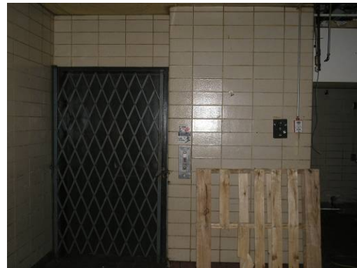
Elevator on 14 th floor
