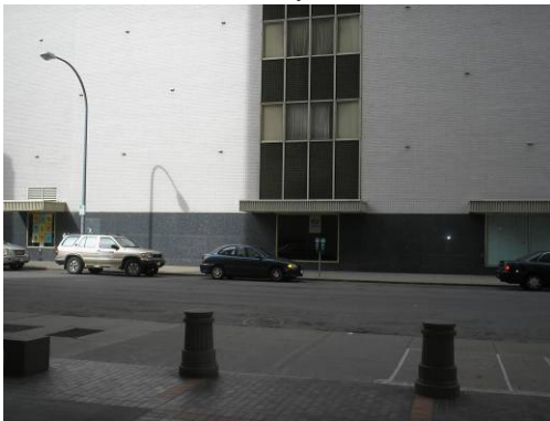
West view of McCurdy's Building
