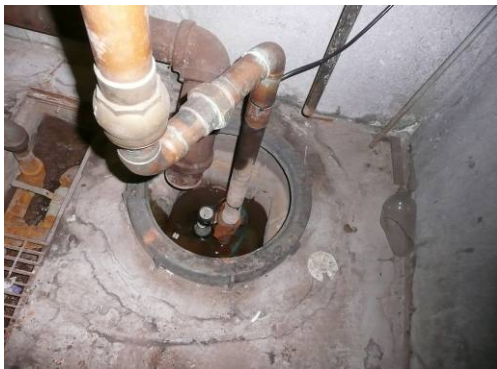
Sump in sub-basement of McCurdy's Building
