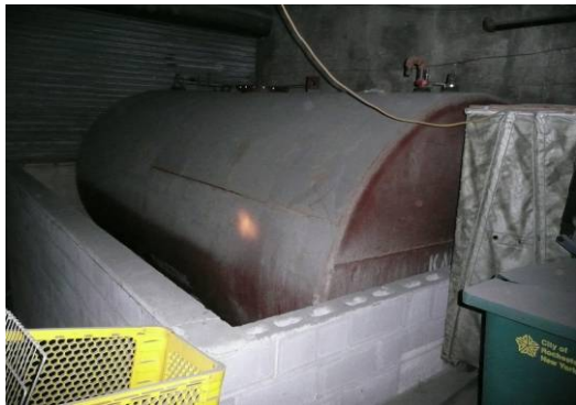
AST in basement of McCurdy's Building
