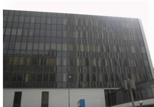
East view of Seneca Building
