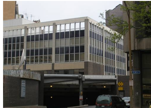
North view of Euclid Building and entrance to underground service tunnel
