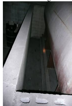
AST in basement of McCurdy's Building
