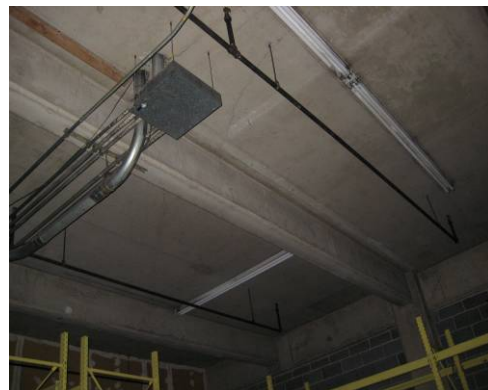
Basement (Room 4) of Seneca Building
