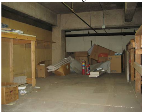
Basement (Room 3) of Seneca Building
