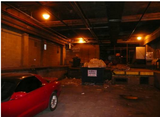
Underground service tunnel near Seneca Building loading dock
