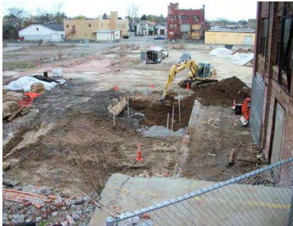
Photo No. 51– AOC-2: Backfilling of northeast corner.
