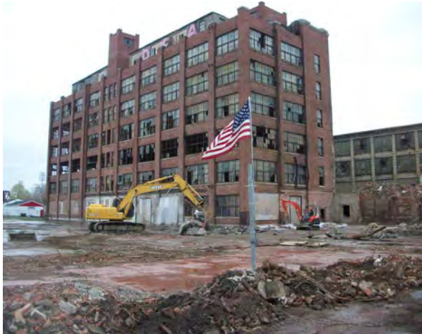
Photo No. 1 – AOC-1 concrete cover removal over UST vault system.
