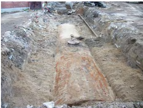
Photo No. 5 – AOC-1: View looking south at exposed 10,000-gal Tank 9.
