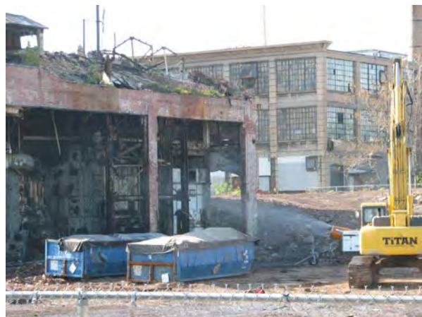
Photo No. 30- View looking south at boiler house demolition activity, 2008.
