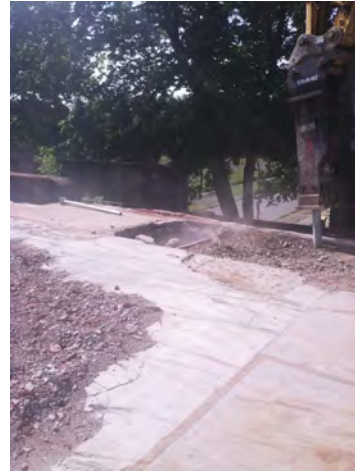
Photo No. 2: Test pit by railroad.
