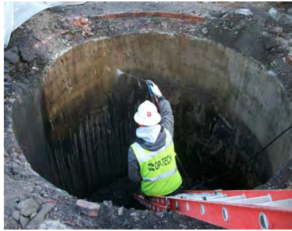
Photo No. 28- AOC-2: OPTECH steam-cleaning interior concrete of chimney.
