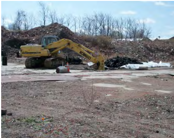
Photo No. 27- AOC-2: Excavator removing building demo debris from chimney.
