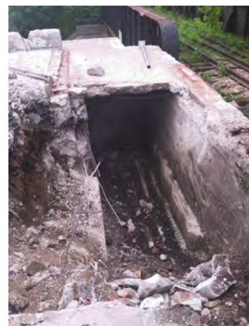
Photo No. 6: Contents of test pit by railroad.
