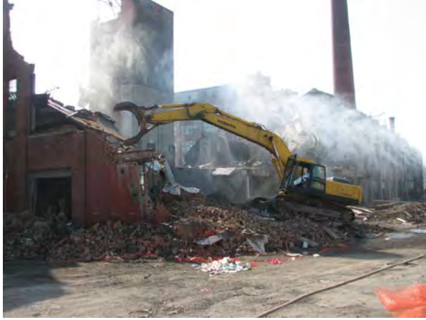
Photo No. 25 – View to south at demolition of 354 Whitney St. building, 2008.
