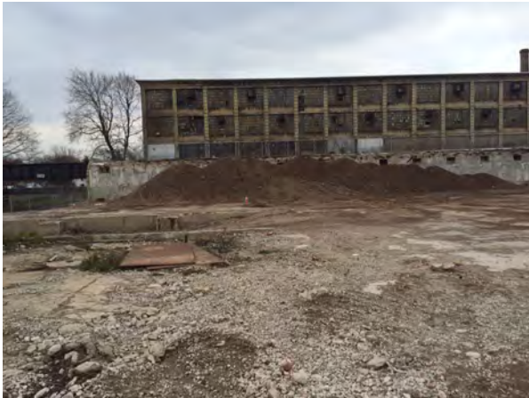
Photo No. 3: Pile Relocation Along South Wall
