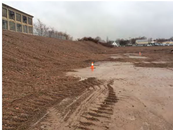
Photo No. 10: Final Berm Built With Building Debris and Dirt
