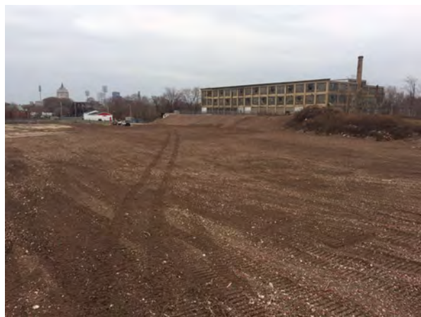
Photo No. 12: Over all grading from NW Corner
