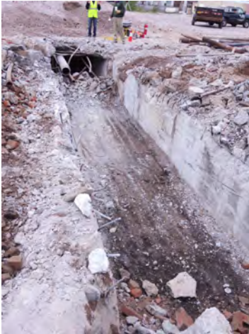
Photo No. 13: Pipe trench with pipes removed.
