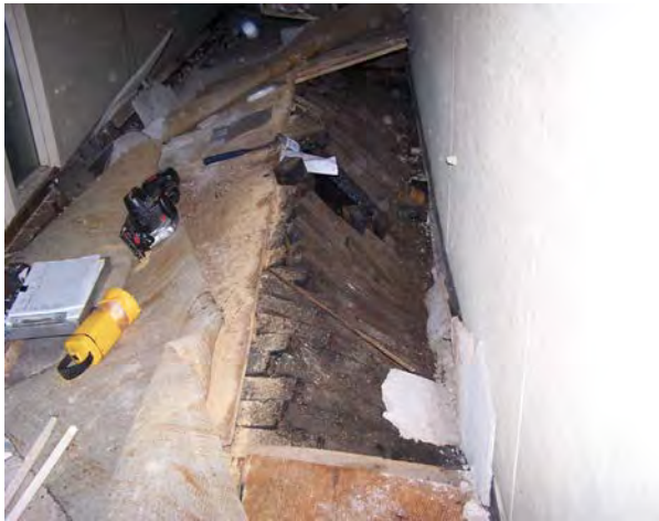
Photo No. 3 – View of treated wood block floor in 415 Orchard St. building, 2006.
