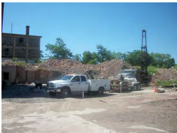
Photo No. 59 – Nothnagle Drilling installing boring PA-18, west of Plating Area, 2011.
