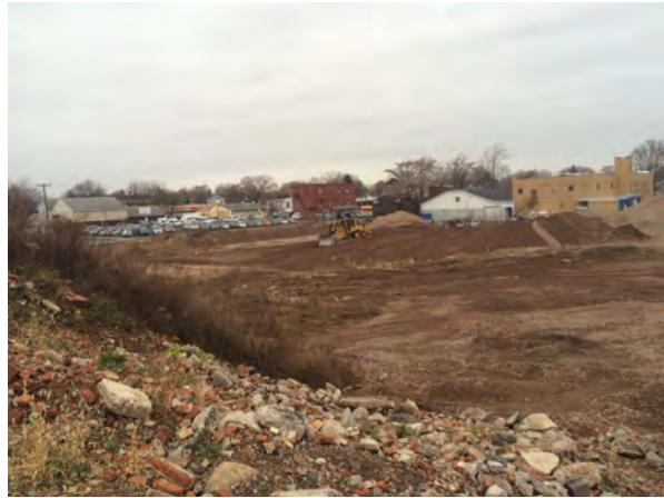
Photo No. 4: Grading In West Side of Lot
