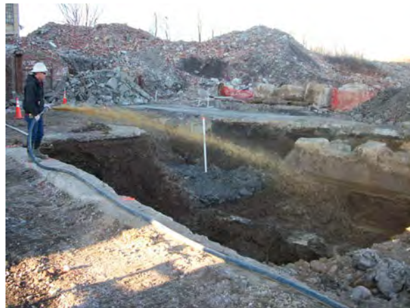
Photo No. 48- AOC-2: Applying molasses remedial agent to open excavation.
