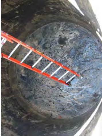
Photo No. 31 – AOC-2: Cleaned chimney base prior to backfilling.
