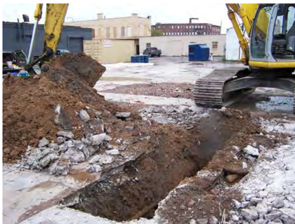
Photo No. 41 – Excavation of TP-03 on north side of hydraulic lift, 2008.
