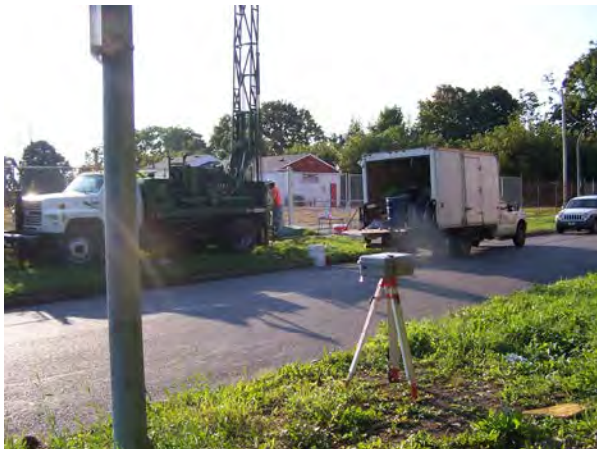
Photo No. 35 – Soil boring SB-03 installation east of Site along Orchard Street, 2008.
