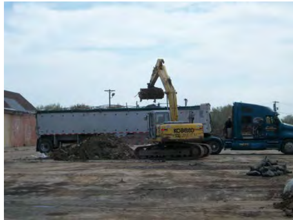
Photo No. 52 – AOC-2: Loading of hazardous soil on Low Rise slab.
