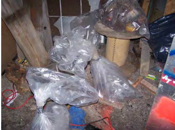
Photo No. 13 – Bagged waste materials during abatement in Low-Rise building, 2008.
