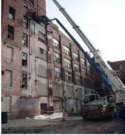
Photo No. 19 – Transformer removal process at 415 Orchard St. building, 2008.
