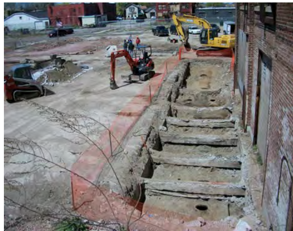
Photo No. 10. - AOC-1: View looking north at exposed tank farm.
