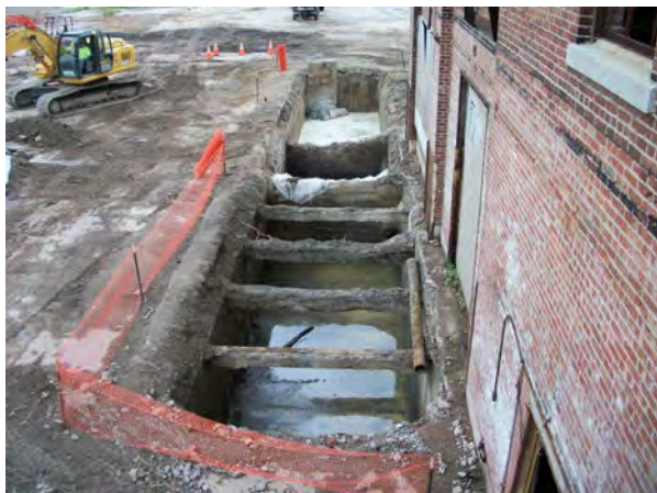
Photo No. 23. – View north at vault cleaned of contaminated bedding material.
