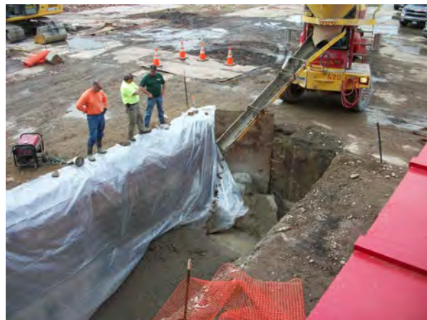
Photo No. 24. – AOC-1: Placing flowable fill in Tank 9 vault.
