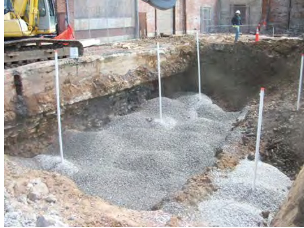
Photo No. 62 – Installation of 2" backfilled wells in former Plating Area, 2012.
