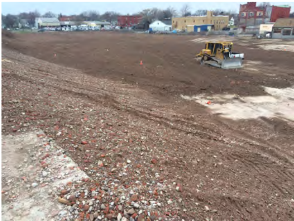
Photo No. 9: Final Berm Built With Building Debris and Dirt
