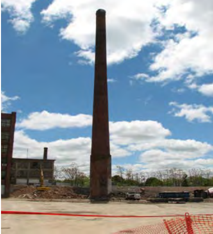
Photo No. 31 – View looking south at chimney after boiler house demolition, 2008.
