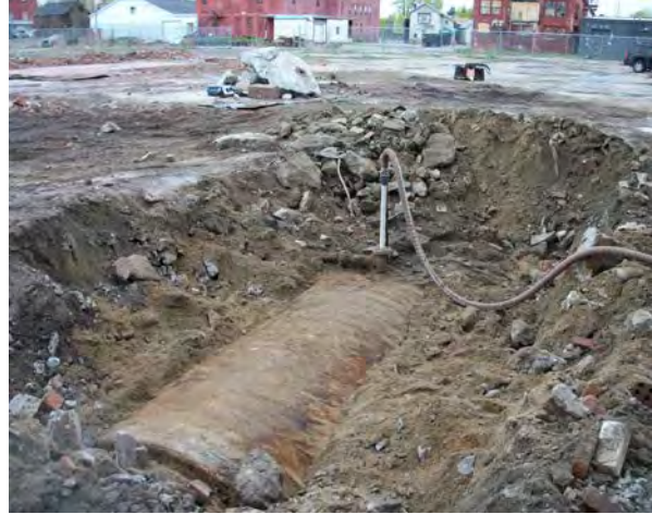
Photo No. 8. – AOC-1: View looking north at product removal in Tank 9.
