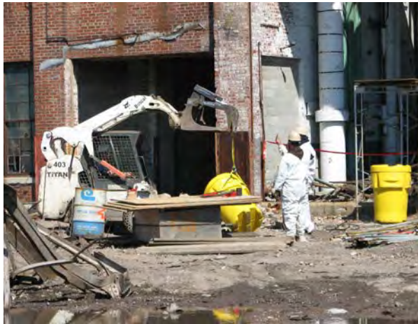
Photo No. 21 – Titan removing over-pack drums of hazardous materials from 354 Whitney St. bldg., 2008.
