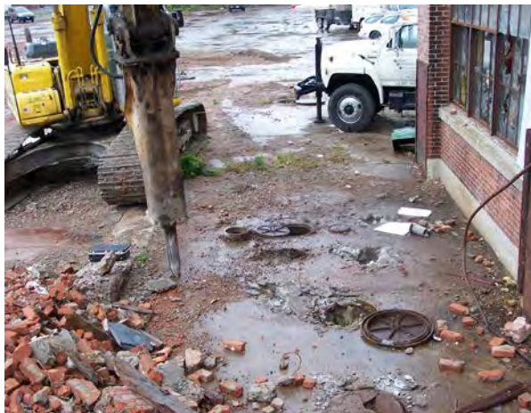
Photo No. 39 – Hoe-ram accessing UST cover system, 2008.
