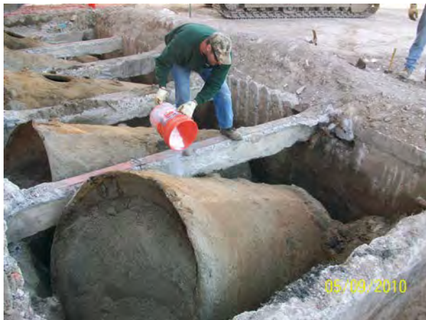
Photo No. 15 – AOC-1: Inerting tank prior to removal.
