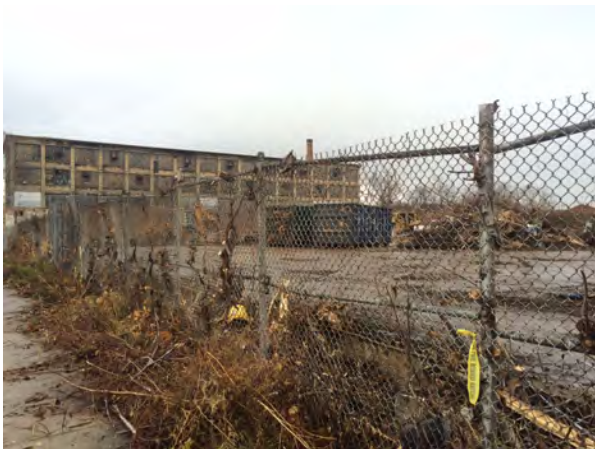
Photo No. 5: Vegetation Clearing
