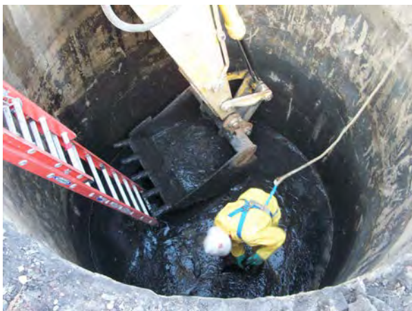
Photo No. 29. – AOC-2:Removal of residual chimney waste liquids.
