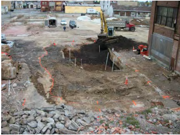
Photo No. 63 – Final backfilling of northeast corner of Plating Area excavation, 2012.
