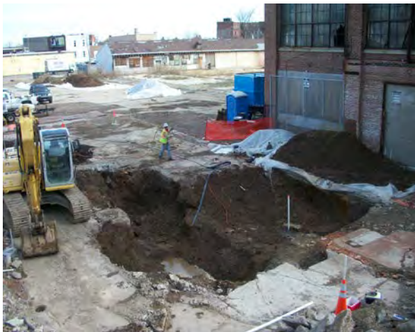
Photo No. 39 – AOC-2: View looking northeast at plating area excavation area.
