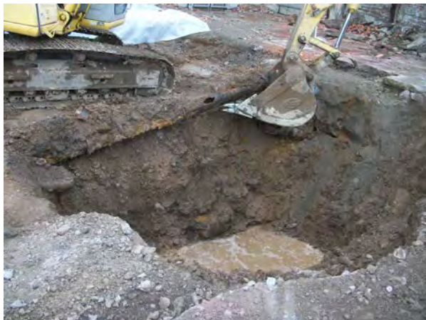
Photo No. 35 – AOC-2: Removal of 8” CI pipe, south-central plating area.
