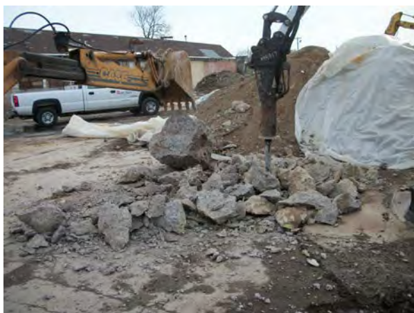
Photo No. 53 – AOC-2: Breaking of chromium contaminated concrete block.
