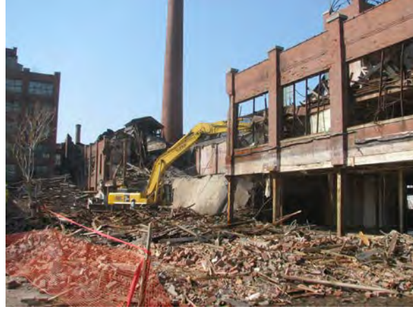
Photo No. 26 – South view of demolition of 354 Whitney St. building, 2008.
