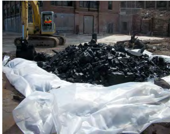
Photo No. 26 –AOC-2: Building demolition debris removed from chimney base.
