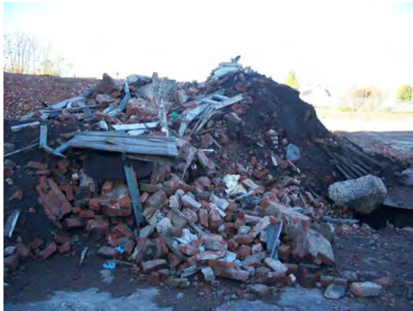
Photo No. 33 – View looking west at chimney ash/debris ready for disposal, 2008.
