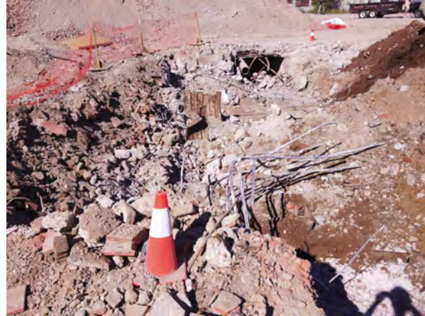
Photo No. 18: Concrete and rebar in the subsurface.
