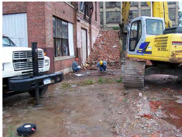
Photo No. 40 – Lu assessing UST system on west side of 415 Orchard bldg., 2008.
