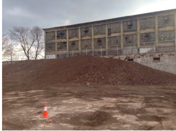
Photo No. 2: Pile Relocation Along South Wall
