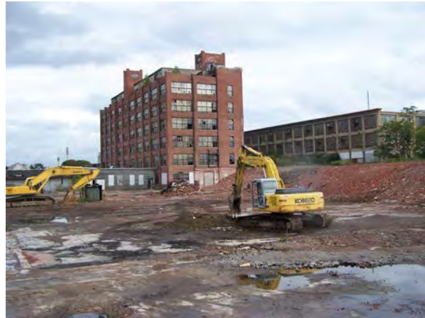
Photo No. 44 – View looking east at excavation of test pits, 2008.
