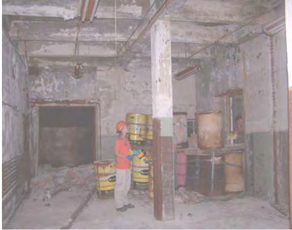
Photo No. 1 – Waste drums stored in tunnel during hazardous materials survey, 2006.
