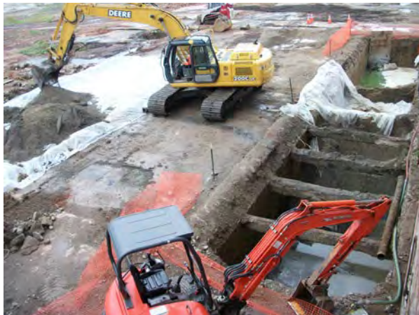
Photo No. 21 – AOC-1: Staging petroleum-impacted sand bedding material.
