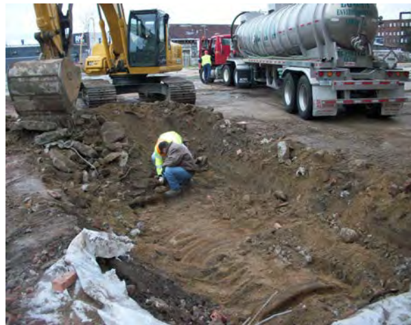
Photo No. 4 – AOC-1: Initial uncovering of 10,000 gal Tank 9.
