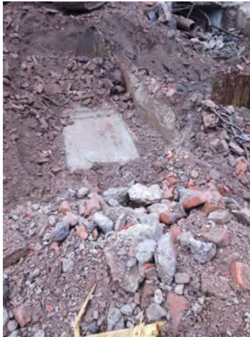
Photo No. 19: Encountered concrete slab.
