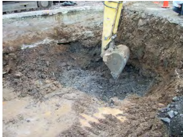
Photo No. 46 – AOC-2: Uncovering petroleum-impacted soil by PA-13.
