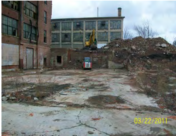
Photo No. 49 – TREC removing bldg demo debris for UST/plating area investigation, 2011.
