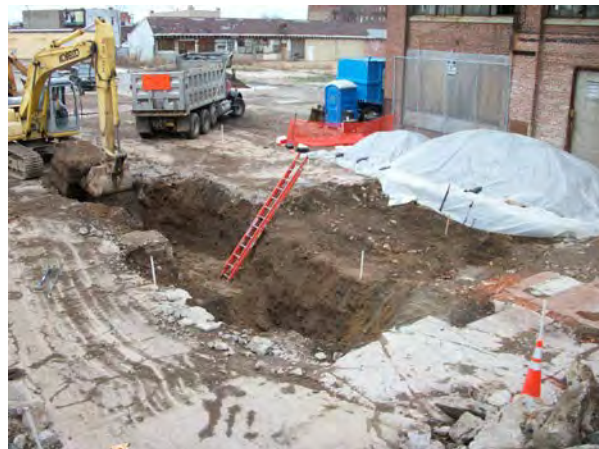
Photo No. 36- AOC-2: Looking northeast at plating area excavation in progress.
