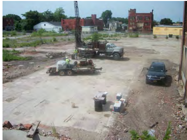
Photo No. 58 – Nothnagle installing Plating Area boring PA-07, 2011.
