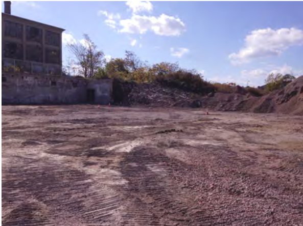
Photo No. 25: Graded Site.
