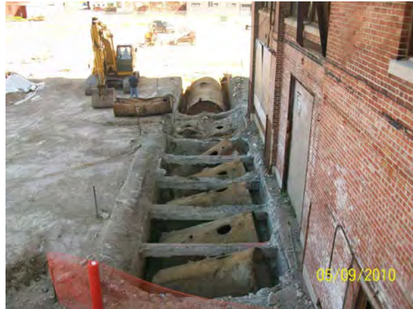
Photo No. 14 – AOC-1: View looking north of tanks ready for removal.
