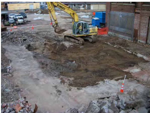
Photo No. 41 – AOC-2: Backfilling southern portion of excavation area.
