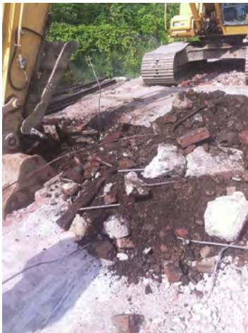
Photo No. 3: Test pit by railroad.
