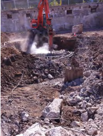
Photo No. 17: Hammering concrete.
