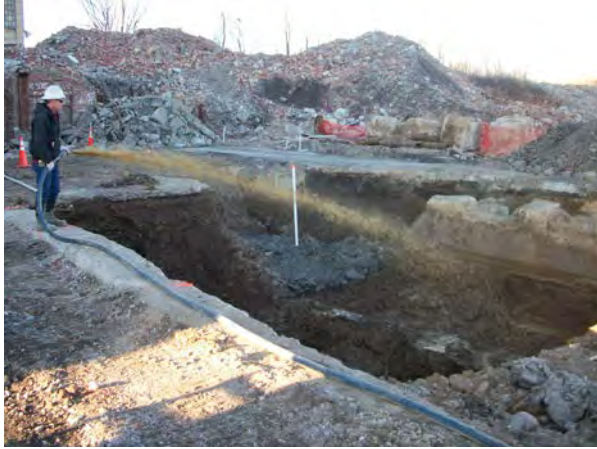
Photo No. 61 – OP-TECH applying molasses solution to Plating Area excavation, 2012.
