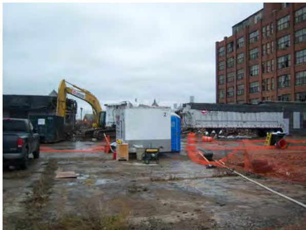
Photo No. 47 – View looking east at Low-Rise demolition activity, 2009.
