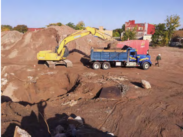
Photo No. 23: Live-loading petroleum impacted soil.
