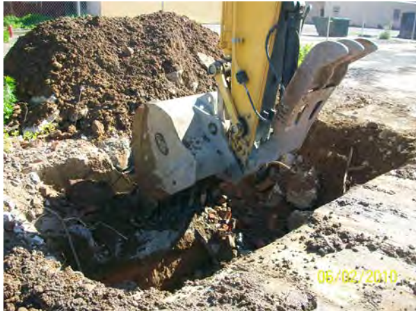
Photo No. 55 – AOC-3: Looking northeast at removal of hydraulic vehicle lift.
