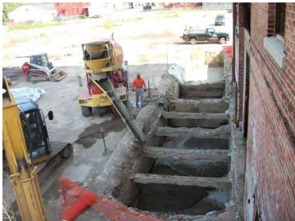
Photo No. 53 – Placing flowable fill in Tank 1-5 vault, 2011.
