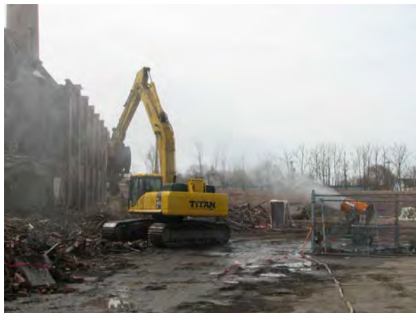
Photo No. 24. – Titan Wrecking demolishing 354 Whitney St. bldg., 2008.
