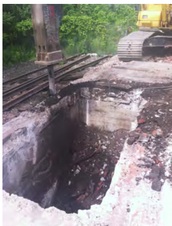
Photo No. 5: Contents of test pit by railroad.
