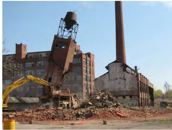
Photo No. 28- View looking south at tower collapse during demolition, 2008.
