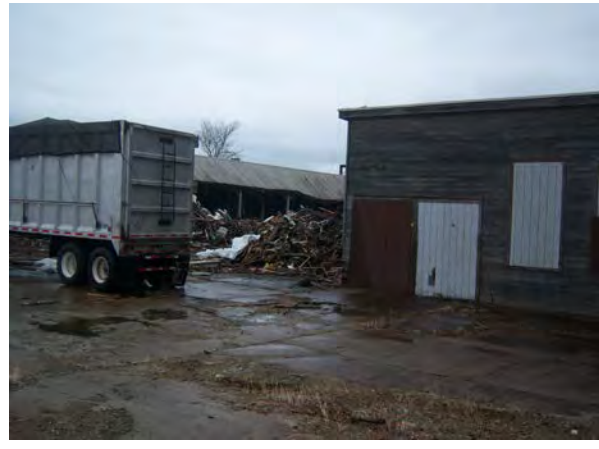
Photo No. 46 – View looking northeast at demolition of Low-Rise structure, 2009.
