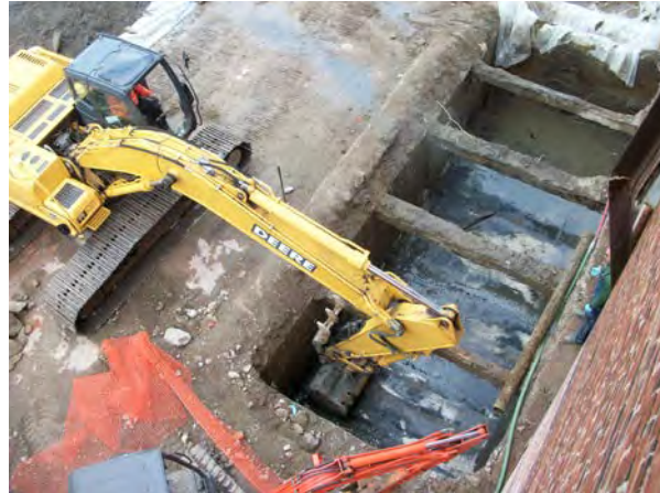
Photo No. 52 – TREC removing sand bedding material for vault inspection, 2011.
