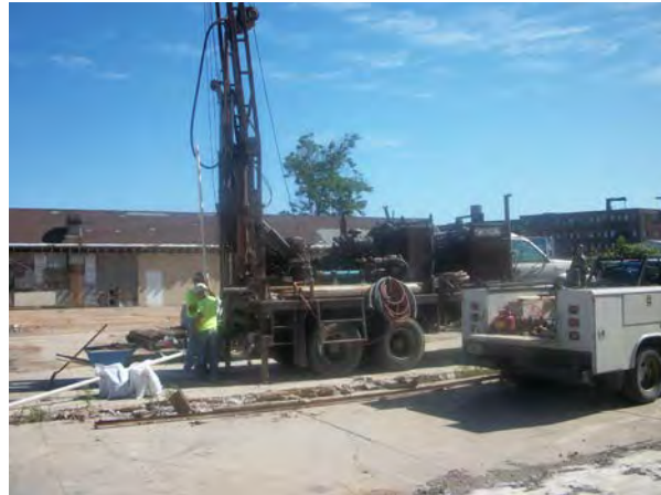
Photo No. 56 – Nothnagle Drilling installing MW-23 in former Low-Rise area, 2011.
