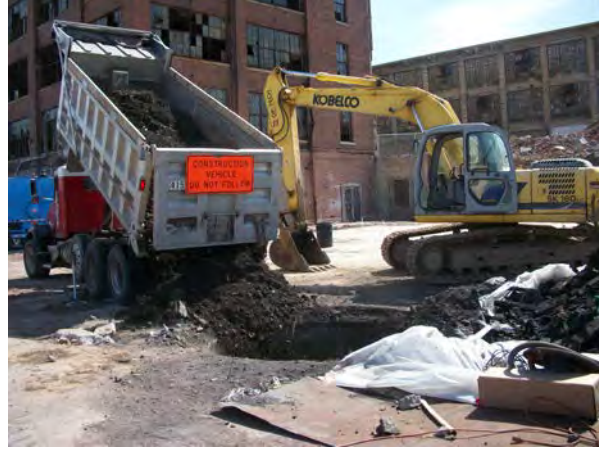
Photo No. 32 – AOC-2: Backfilling of chimney base with site-derived backfill.
