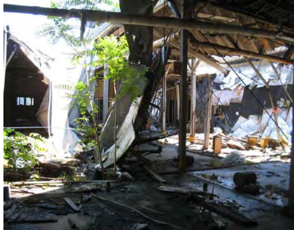
Photo No. 8. – Interior of Low-Rise building, 2006.
