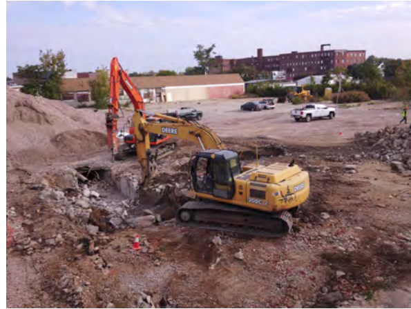
Photo No. 14: Hammer and excavation overview.
