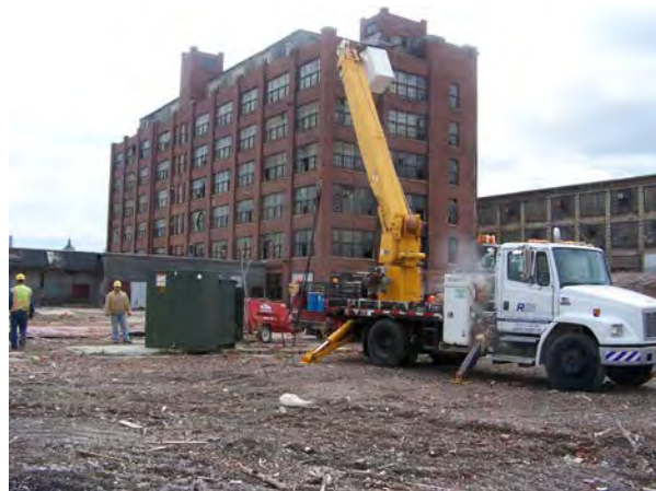
Photo No. 48 - RG&E removing electrical transformer from center of Site, 2009.
