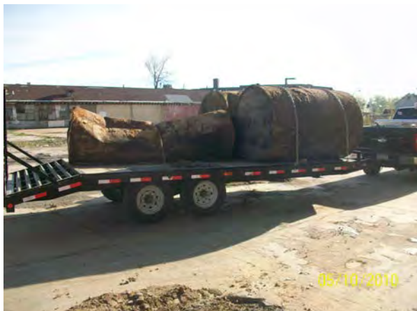
Photo No. 17 – AOC-1: Tank 6, 7 and 8 ready for disposal as scrap metal.
