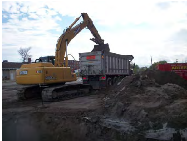
Photo No. 22. – AOC-1: TREC loading petroleum-contaminated sand bedding.
