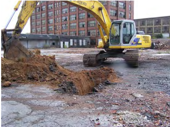
Photo No. 43 – View looking southeast while excavating test pit TP-08, 2008.
