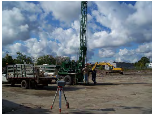
Photo No. 34 – View looking southwest at installation of soil boring SB-20, 2008.
