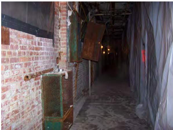
Photo No. 15 – View of asbestos abatement tent in 354 Whitney St. building, 2008.
