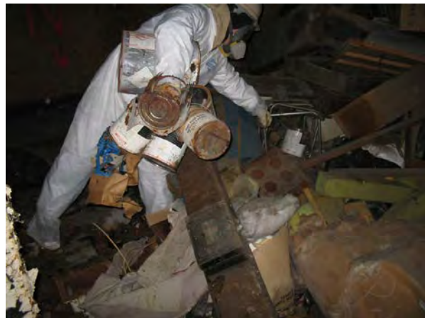
Photo No. 16 – Hazardous material removal in 354 Whitney St. building, 2008.
