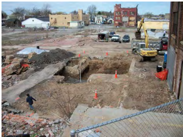
Photo No. 47 – AOC-2: Looking north at plating area excavation overview.
