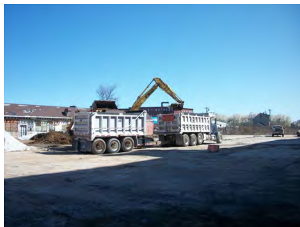
Photo No. 54- AOC-2: Loading of non-hazardous soil from plating area.
