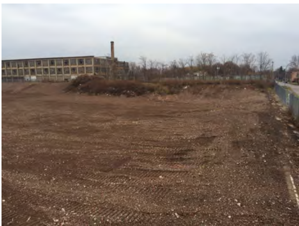
Photo No. 11: Over all grading from NE Corner
