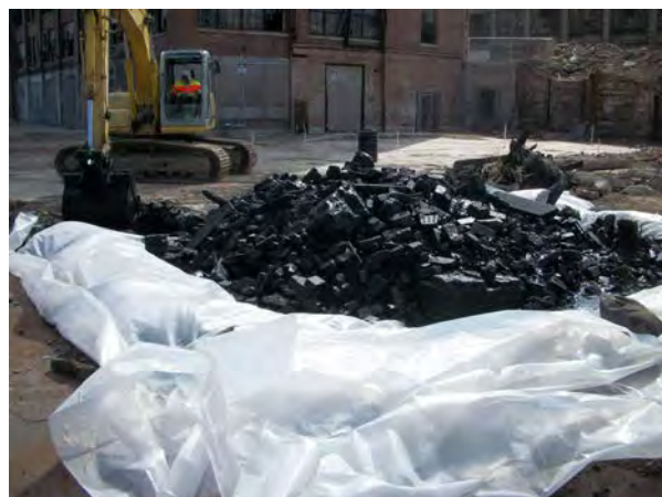
Photo No. 60 – Removing/staging chimney debris (Plating Area wells in background), 2012.
