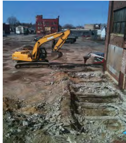
Photo No. 50 – TREC removing concrete cover & exposing UST vault system, 2011.
