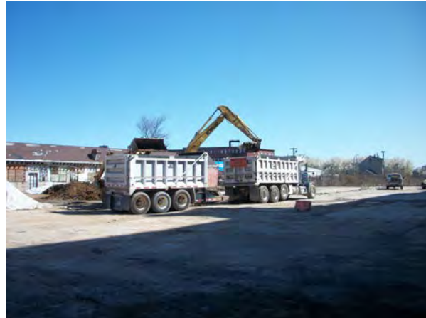
Photo No. 64 – OP-TECH loading contaminated soil into truck for off-site disposal, 2012.
