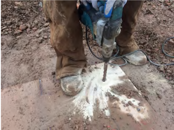
Photo No. 7: Plate Cover Installment
