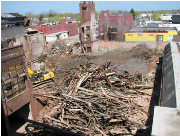
Photo No. 27 – View looking north at building demolition & material segregation, 2008.
