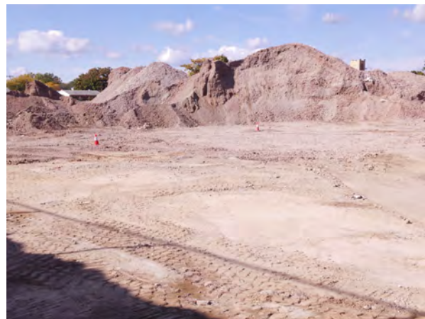
Photo No. 28: Graded Site.
