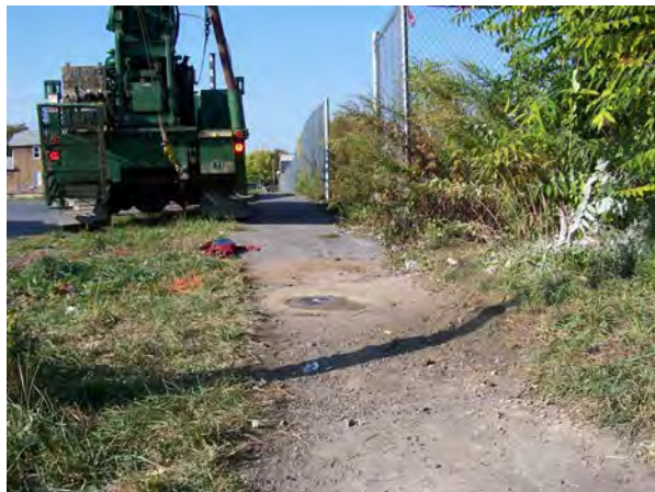
Photo No. 36 - Completion of MW-9 in Whitney Street sidewalk, 2008.
