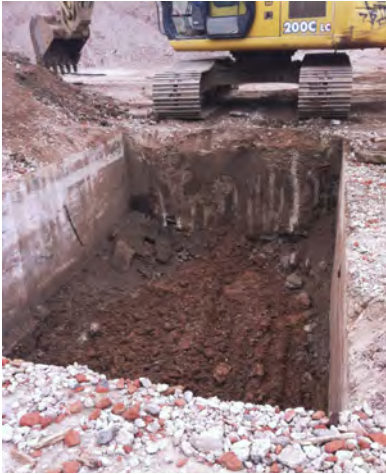
Photo No. 7: Former freight elevator shaft.
