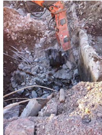
Photo No. 20: Continued concrete hammering.
