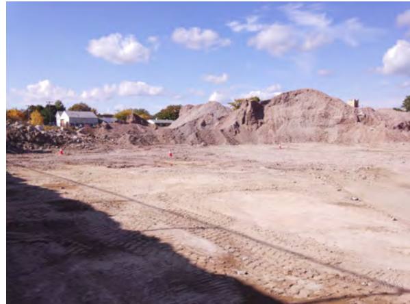
Photo No. 26: Graded Site.
