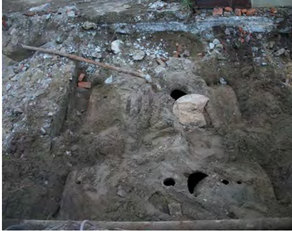
Photo No. 7. – AOC-1: View looking east at Tank 7 & Tank 8.
