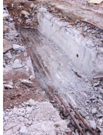
Photo No. 12: Pipe trench with pipes removed.
