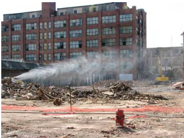
Photo No. 29. – View south at dust suppression measures during demolition, 2008.
