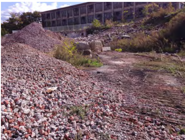
Photo No. 27: Void spaces filled with existing on-site crushed rubble material.
