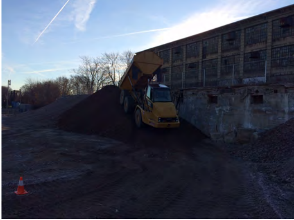
Photo No. 1: Pile Placement Along Wall
