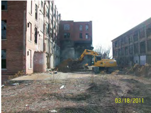
Photo No. 55 – View looking east at excavation of test pit TP-25, 2011.
