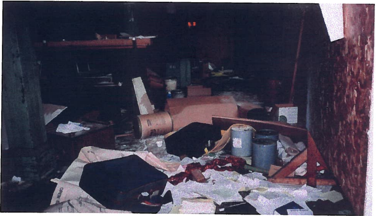
354 Whitney Street; typical debris and containers in building
