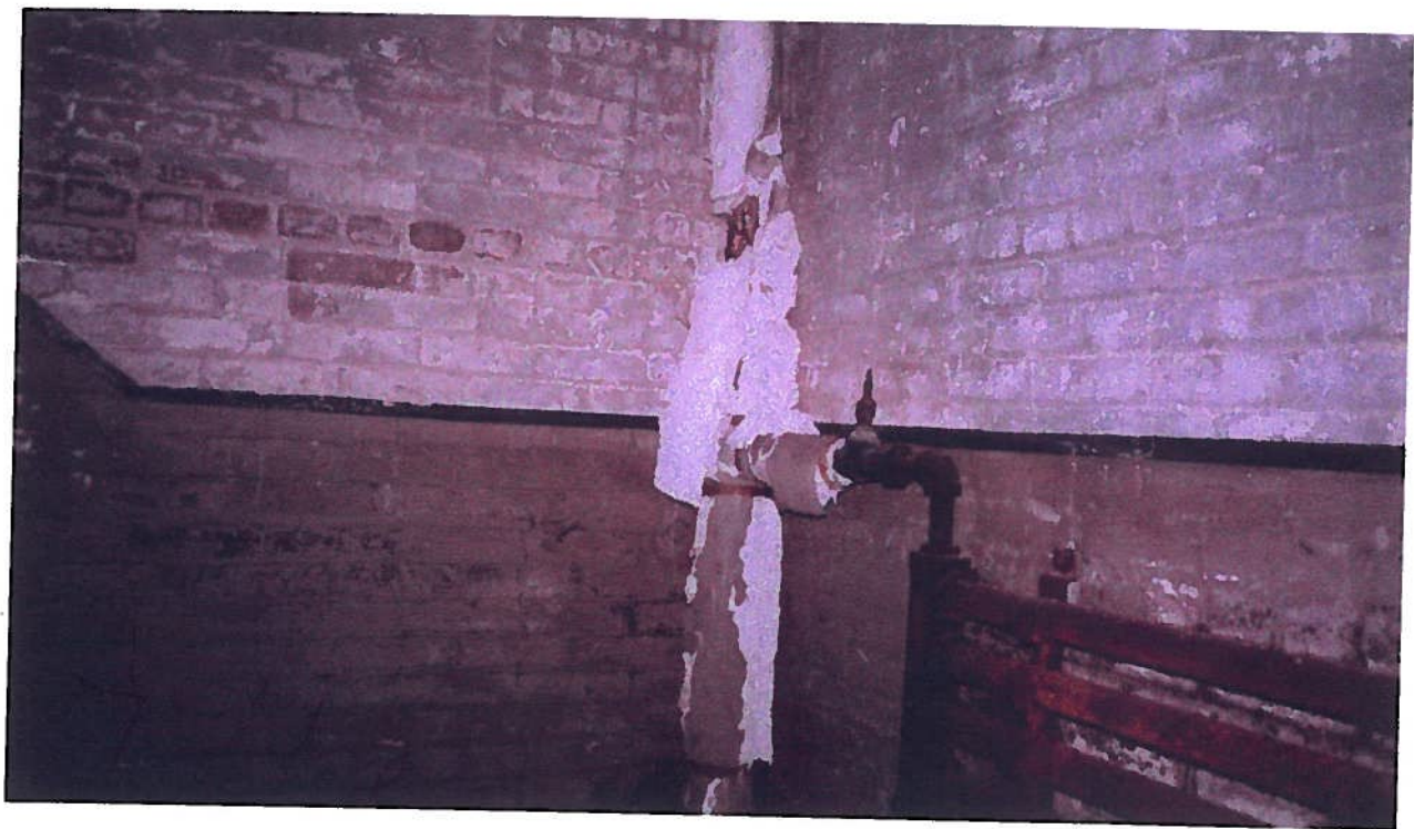
354 Whitney Street; damaged suspect asbestos-containing material in staircase
