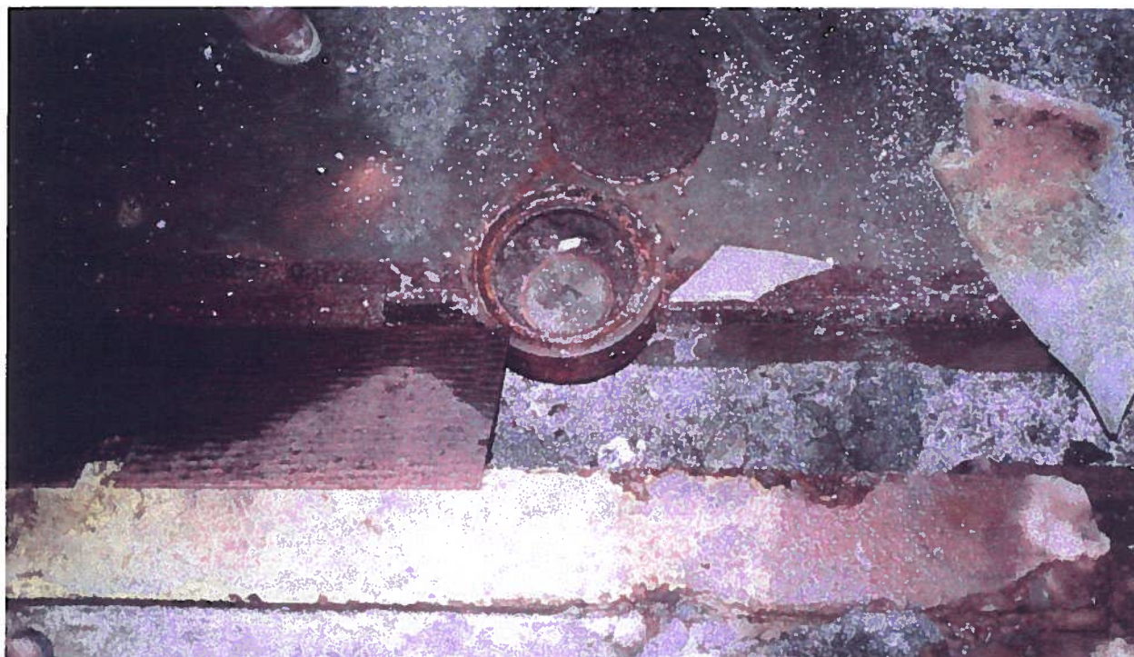
415 Orchard Street; trench drain location ✓
