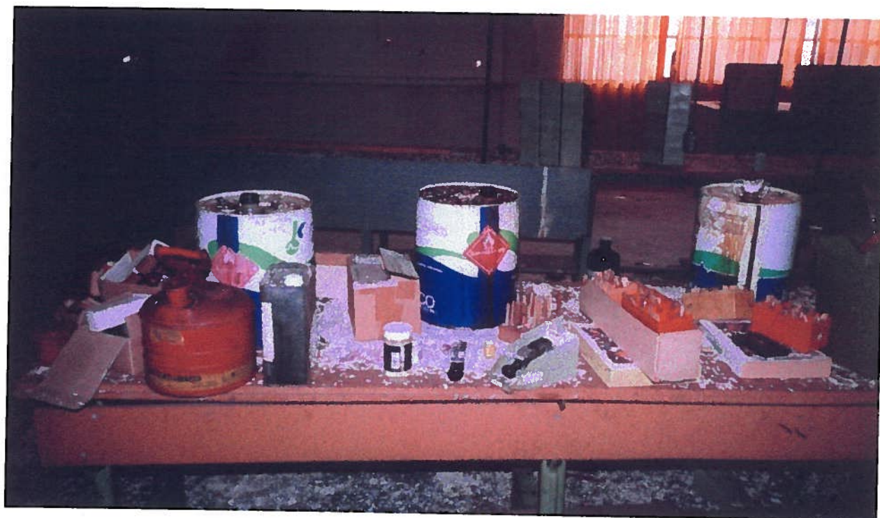
367 Orchard Street; containers of chemicals on 3 rd floor
