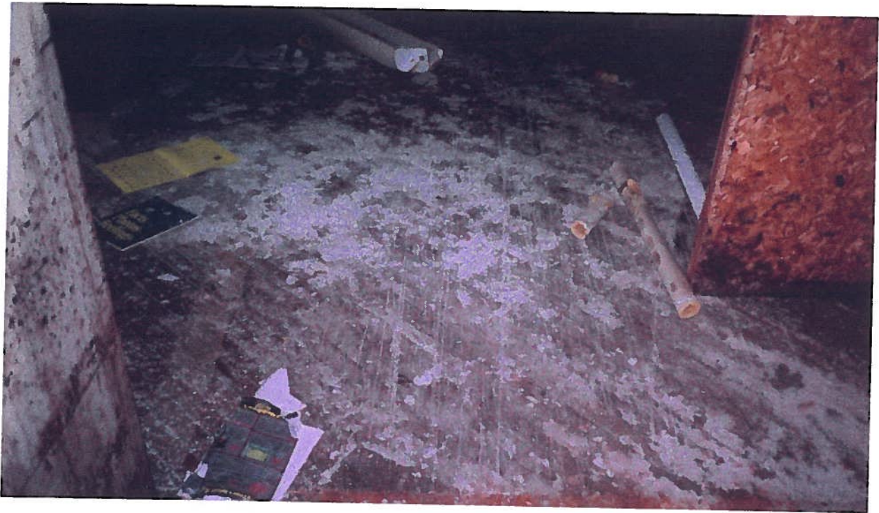
354 Whitney Street; blanketing material determined to be asbestos-containing material on floor beneath HVAC system
