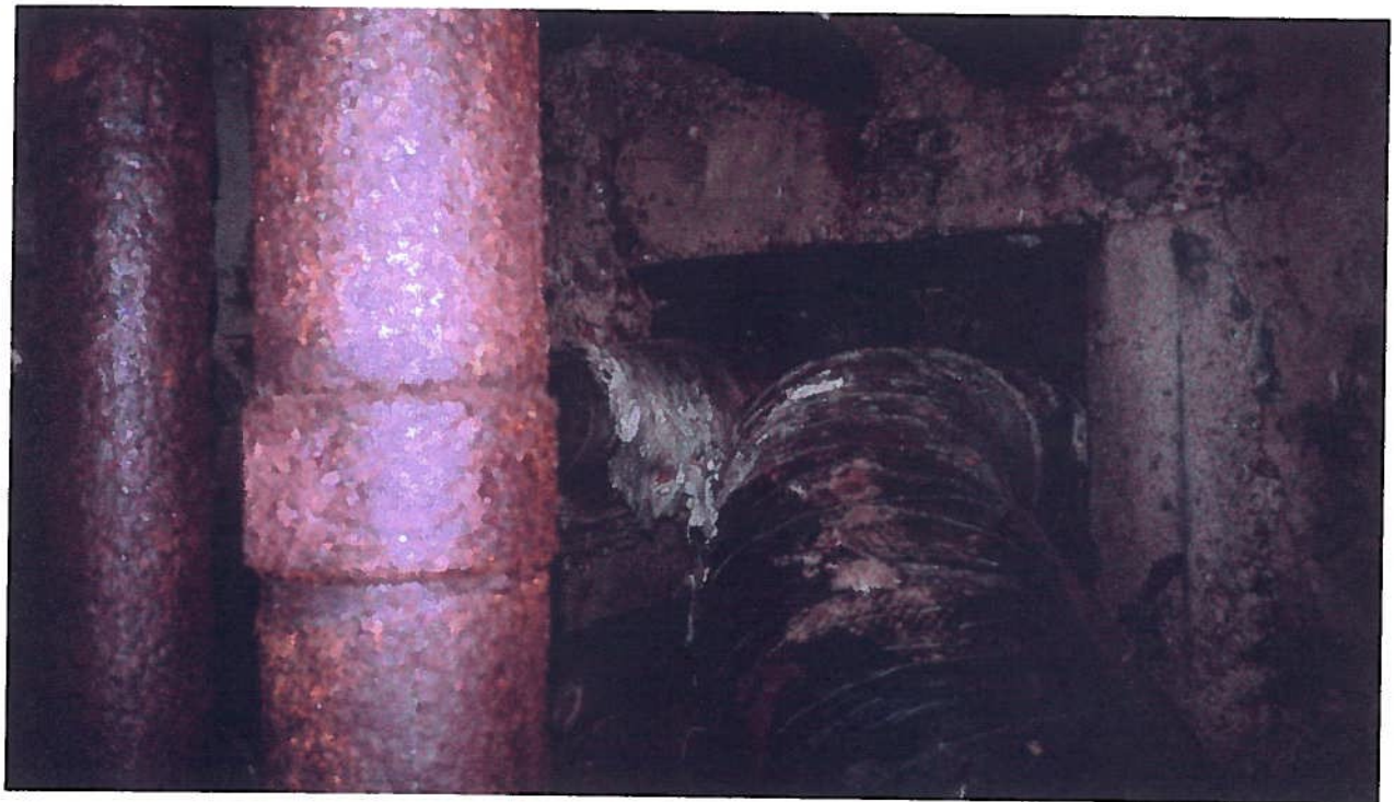
354 Whitney Street; suspect asbestos-containing material located south of boiler room
