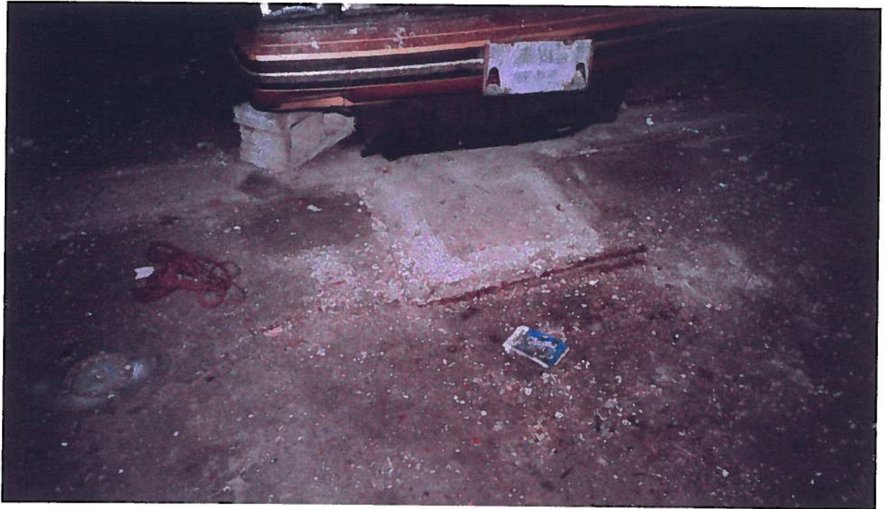
406 Orchard Street; apparent filled-in floor/trench drains and capped floor drain
