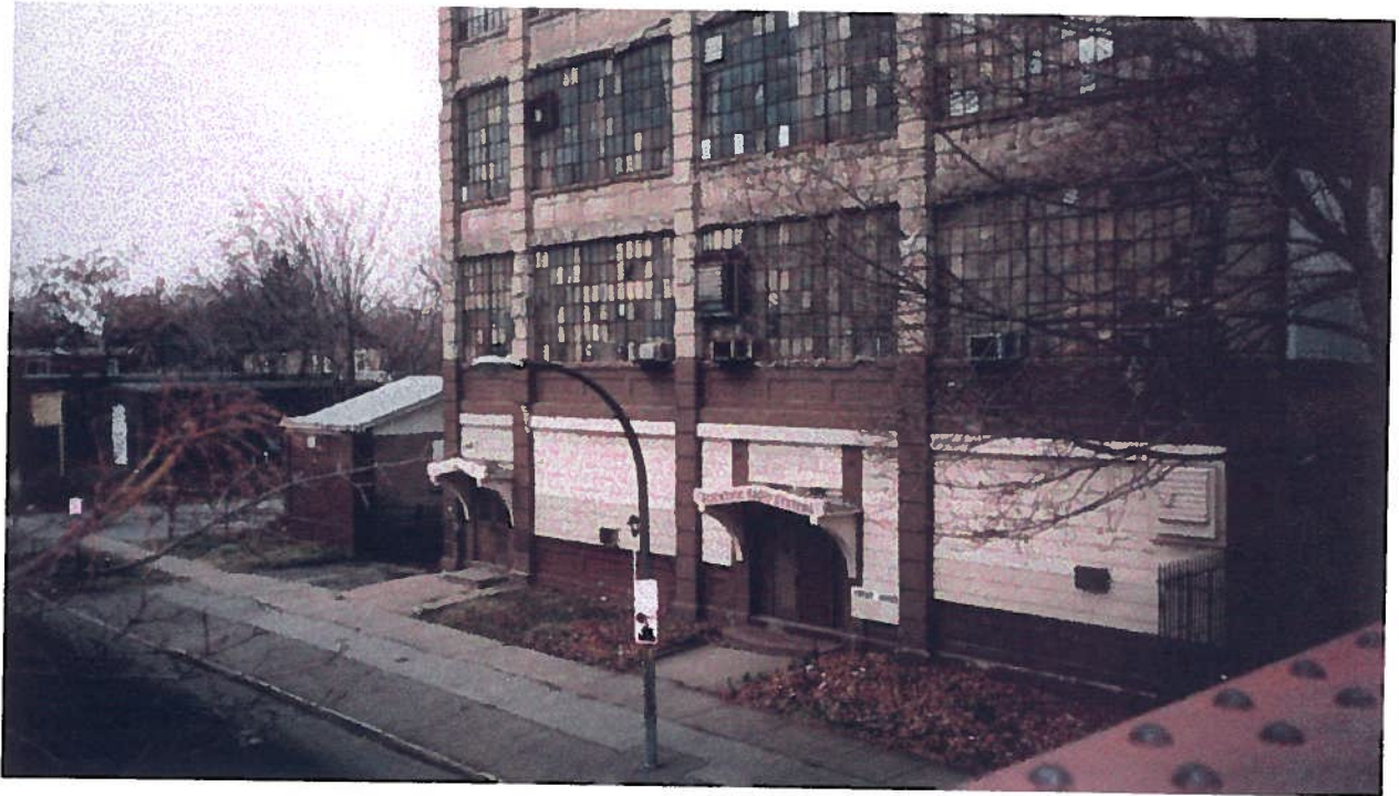
View of 367 Orchard Street looking southwest
