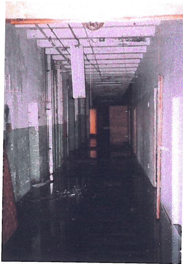
354 Whitney Street; view of water-damage in west wing of building
