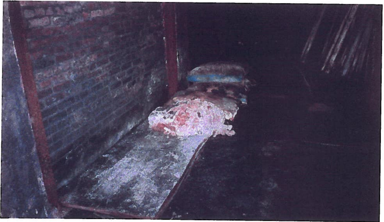
354 Whitney Street; bags labeled as containing light soda ash located southeast/south of the boiler room
