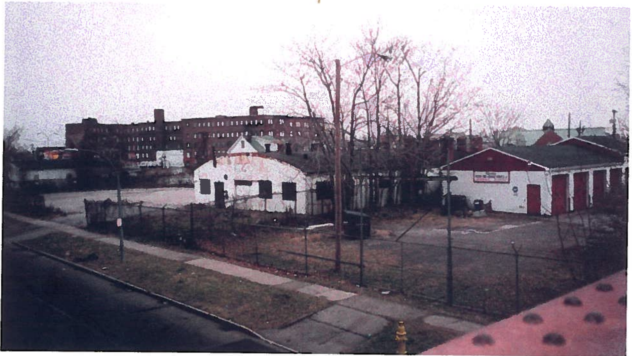
View of 406 Orchard Street looking northeast
